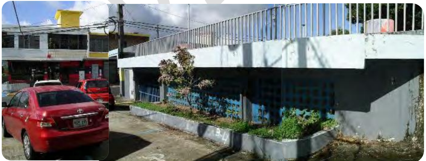
SOUTH - RAISED LEVEL OF PLAZA AND ENTRANCE TO UNDERGROUND PARKING
