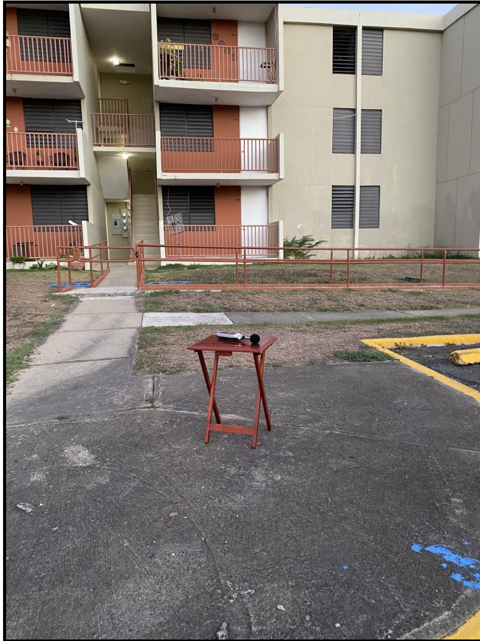
Figure #7- Monitoring Stations #3 location (South Side).
