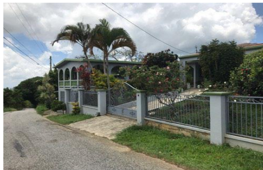
Figure 3. Image of the applicant's house on the property and front gate entrance, view to the northwest.
