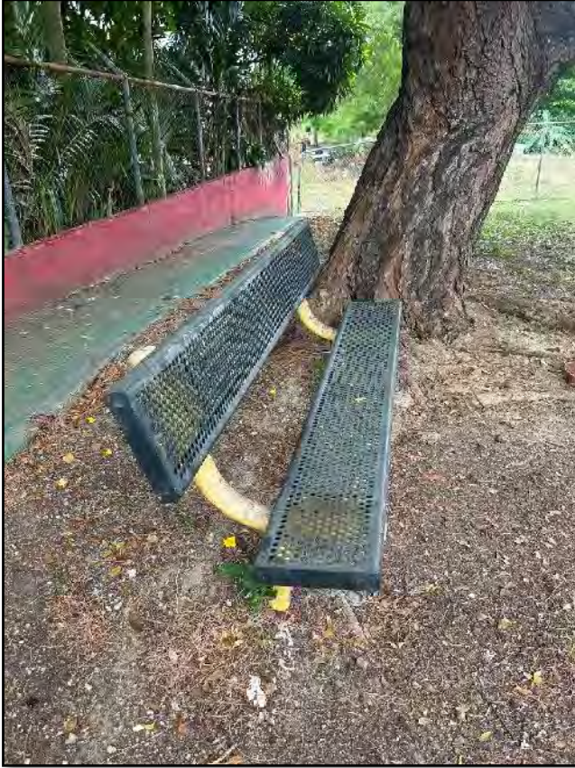
LBP Yellow Metal Bench Support, South Park
