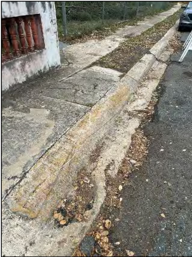
LBP Yellow Concrete Curb, State Road PR-115
