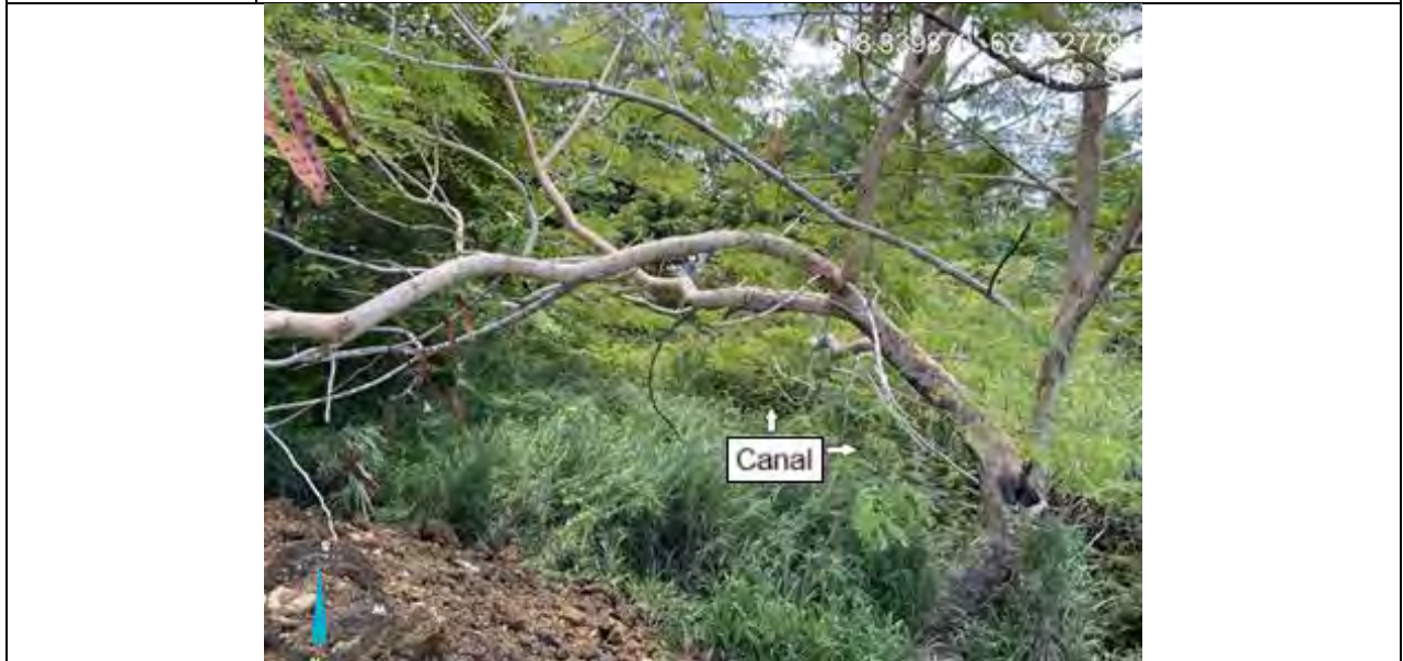
Photo #: 28 Description (South): View of the project area's northern northern perimeter from the neighboring lot. The Ojo de Agua canal can be seen through the vegetation flowing from east to northwest. Date: 7/24/24
