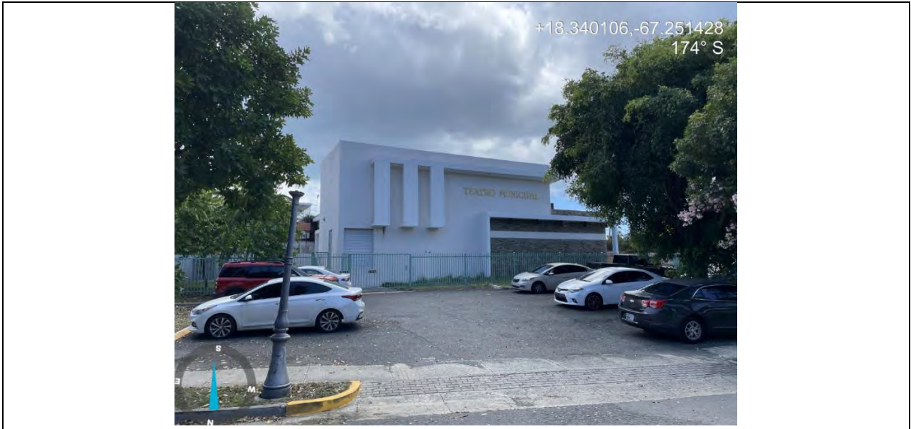
Photo #: 23 Description (South): Rear view of the Rincón Municipal Theater and a section of the municipal parking lot. Both properties are divided by a metal fence. Date: 7/24/24
