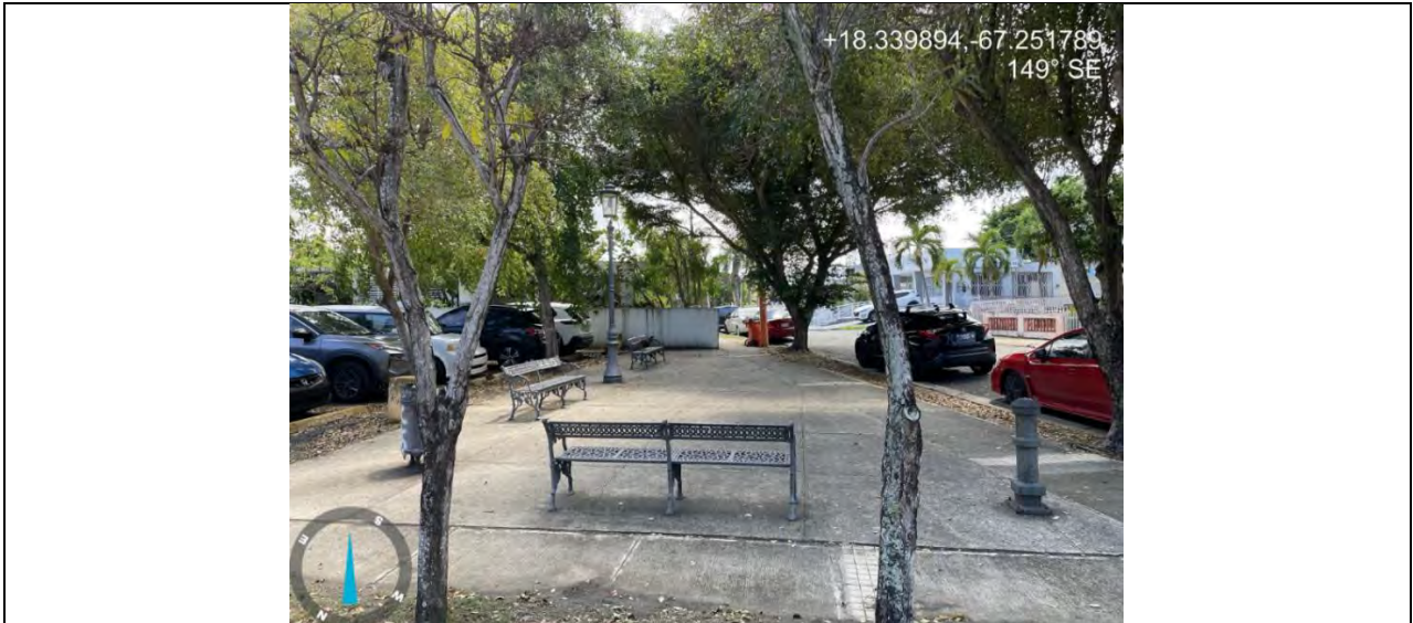
Photo #:25 Description (Southeast): View of park located on the southwest corner of the municipal parking lot (within the project perimeter). The recreation space has a concrete floor and benches, a trash bin, a lamp post and a bollard (all made of metal). Date: 7/24/24
