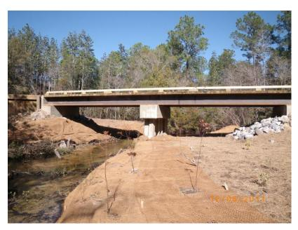
Figure 3. Bridge with Floodplain and Height Capacity for 100 yr Flows.
