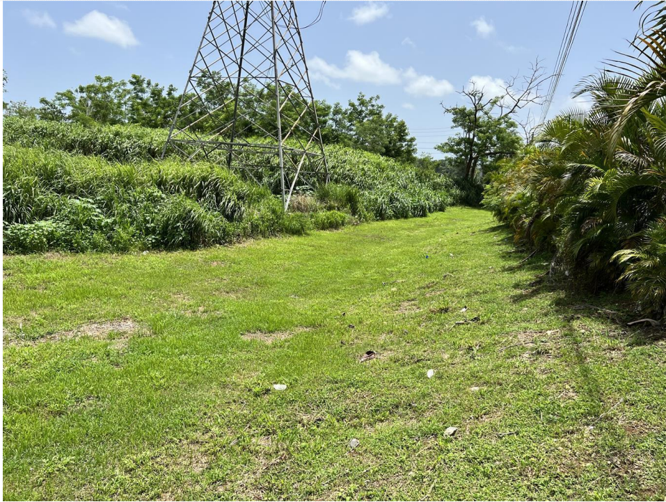
Photo No. 4 Electrical Tower lines north of PR-2. No wetland indicators.
