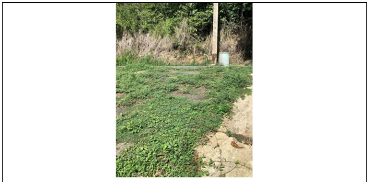
Photo #: 3 Description (include direction): General area where the electrical connection will be installed, looking southwest. Date: September 6 2023
