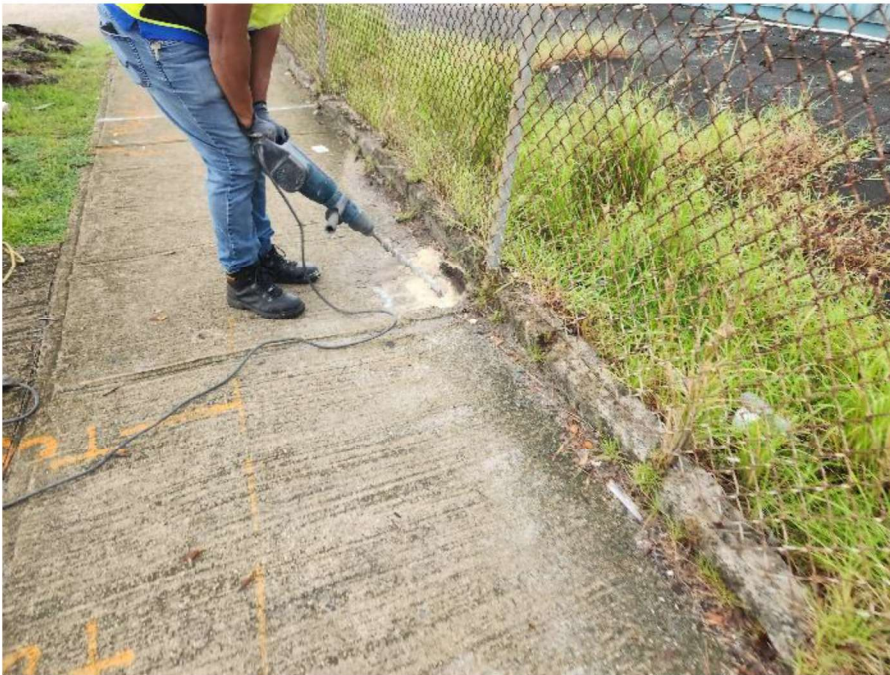
Photograph 4: Concrete breaking at SB-1.
