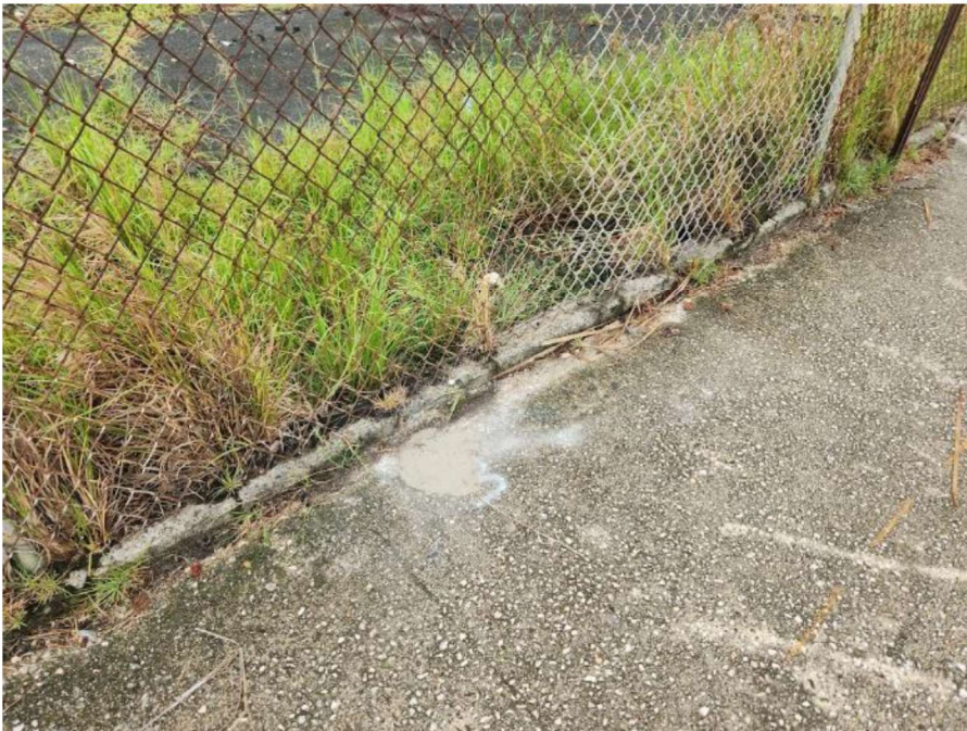
Photograph 30: Cement grouted at SB-3.
