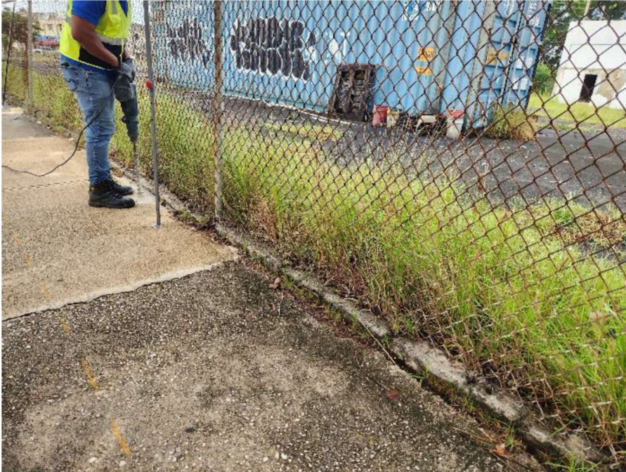
Photograph 7: Concrete breaking at SB-2.
