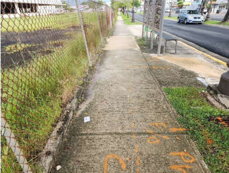
Photograph 1: Underground utilities marked in the area (see yellow lines)
