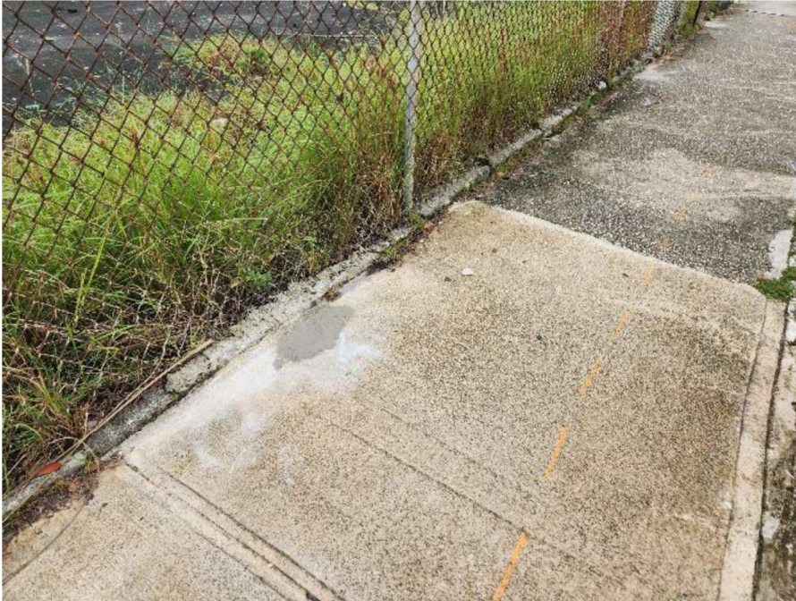
Photograph 29: Cement grouted at SB-2.
