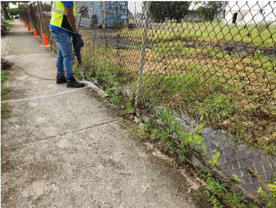
Photograph 16: Concrete breaking at SB-5.
