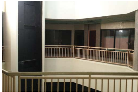
Interior View of the Existing Building
