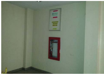
Interior View of the Existing Building
