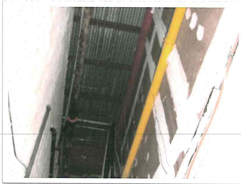
Gas pipeline (yellow) – track aerial at back side corridor POSITIVE to Lead Based Paint
