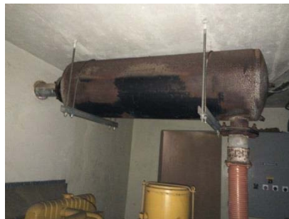
Interior View of the Existing Building
