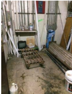
Pails of paint and unidentified liquids, and building materials in a room inside the Building
