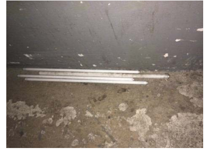
Lamp Ballasts in the interior of the Building
