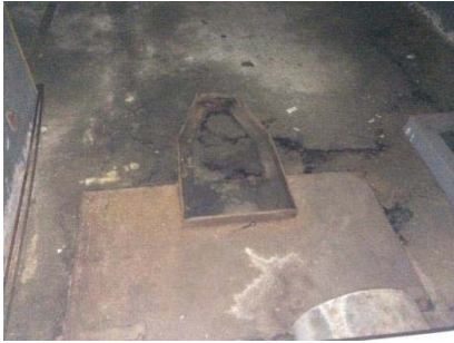
Area used to store garbage
