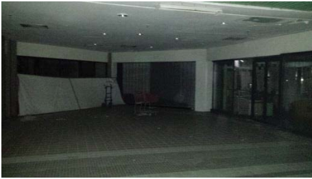
Interior View of the Existing Building
