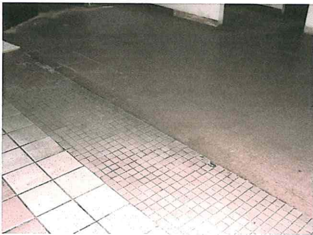
Areas with Vinyl Floor Tiles NEGATIVE to asbestos
