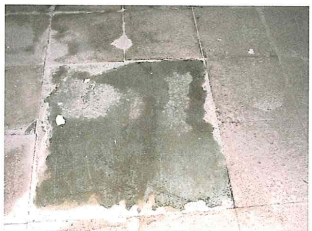
Vinyl Floor Tiles and mastic NEGATIVE to asbestos
