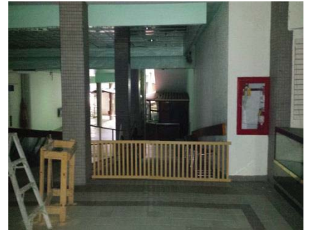
Interior View of the Existing Building
