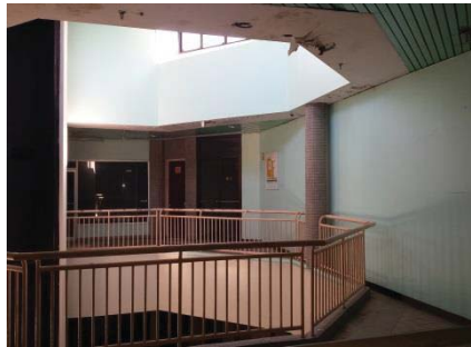
Interior View of the Existing Building
