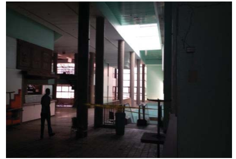
Interior View of the Existing Building
