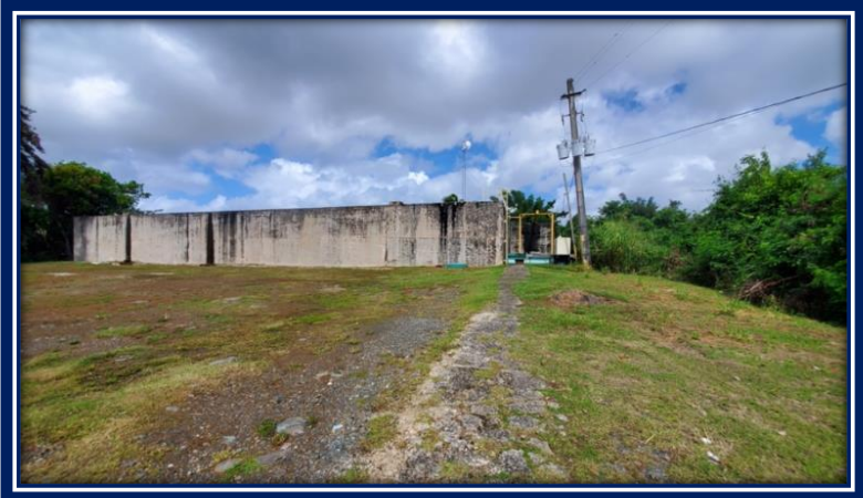
Puerto Rico Aqueduct and Sewer Authority (“PRASA”) – Water Tank
