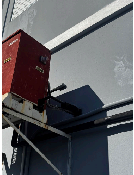
Condensing unit to be replaced (Connections)
