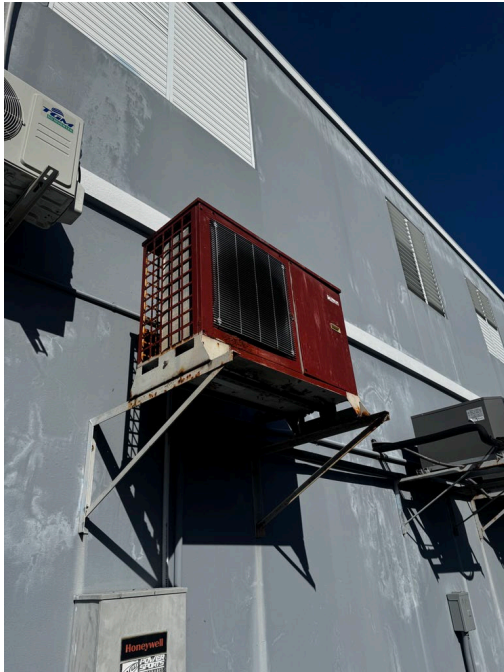
Condensing unit to be replaced
