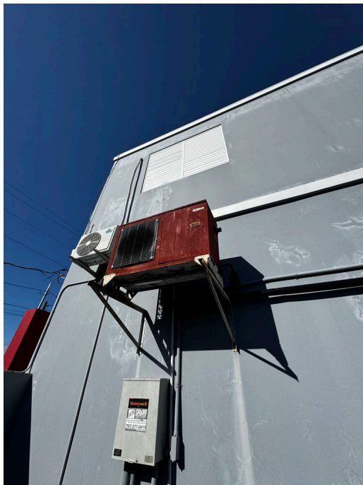
Condensing unit to be replaced (Connections (Better View at the Right Side of Property Photos))
