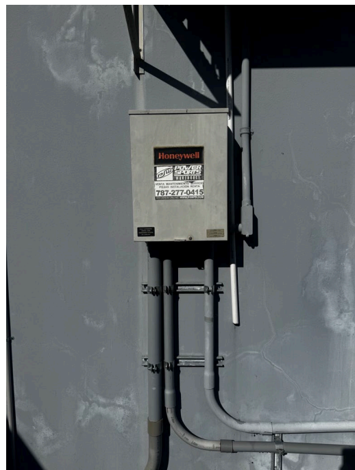
Transfer Switch to be replaced | Right Side of the Property
