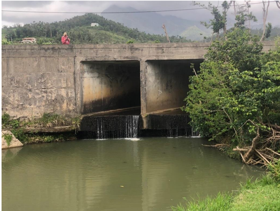
Figure 5. Poor design has resulted in scour and degradation below culvert and obstruction to fish passage.
