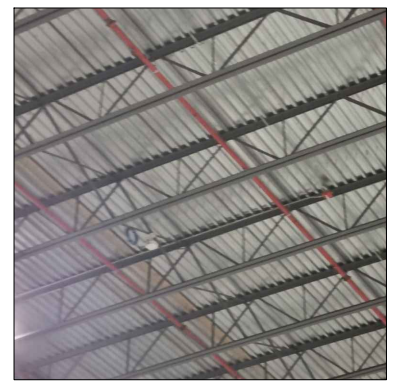
Construction roof support
