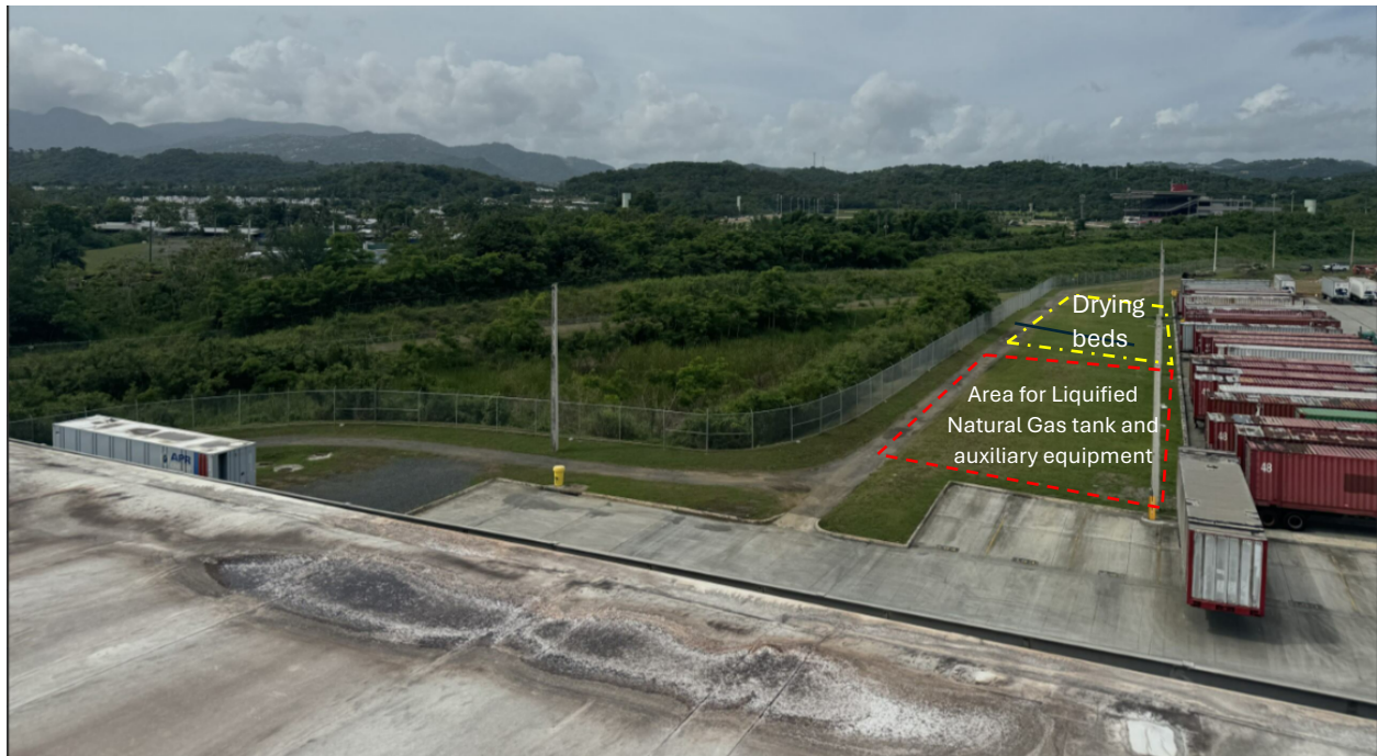
Photo showing the areas where Liquefied Natural Gas (LNG) tank and equipment and drying beds. will be installed
