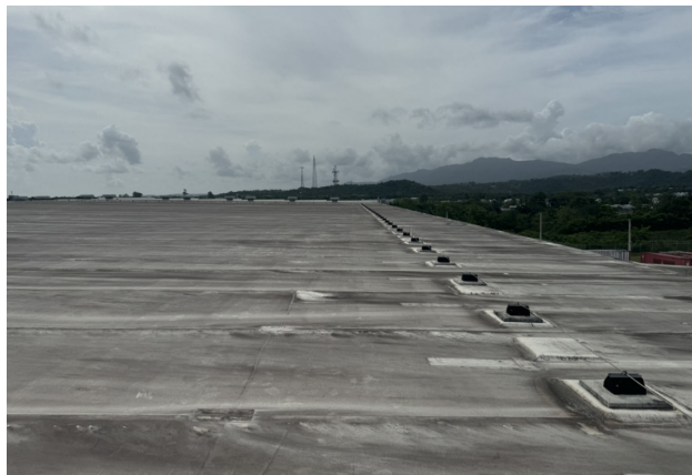
Rooftop where PV panels will be installed
