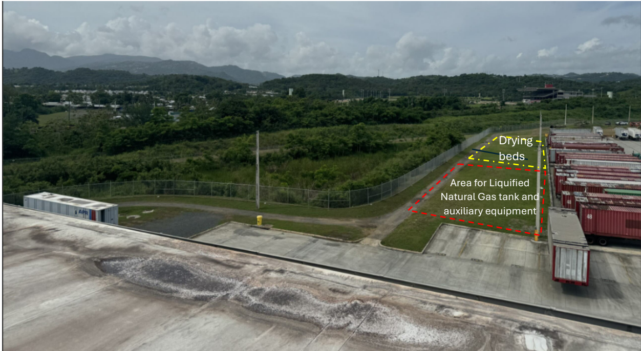
Photo showing the areas where Liquefied Natural Gas (LNG) tank and equipment and drying beds. will be installed
