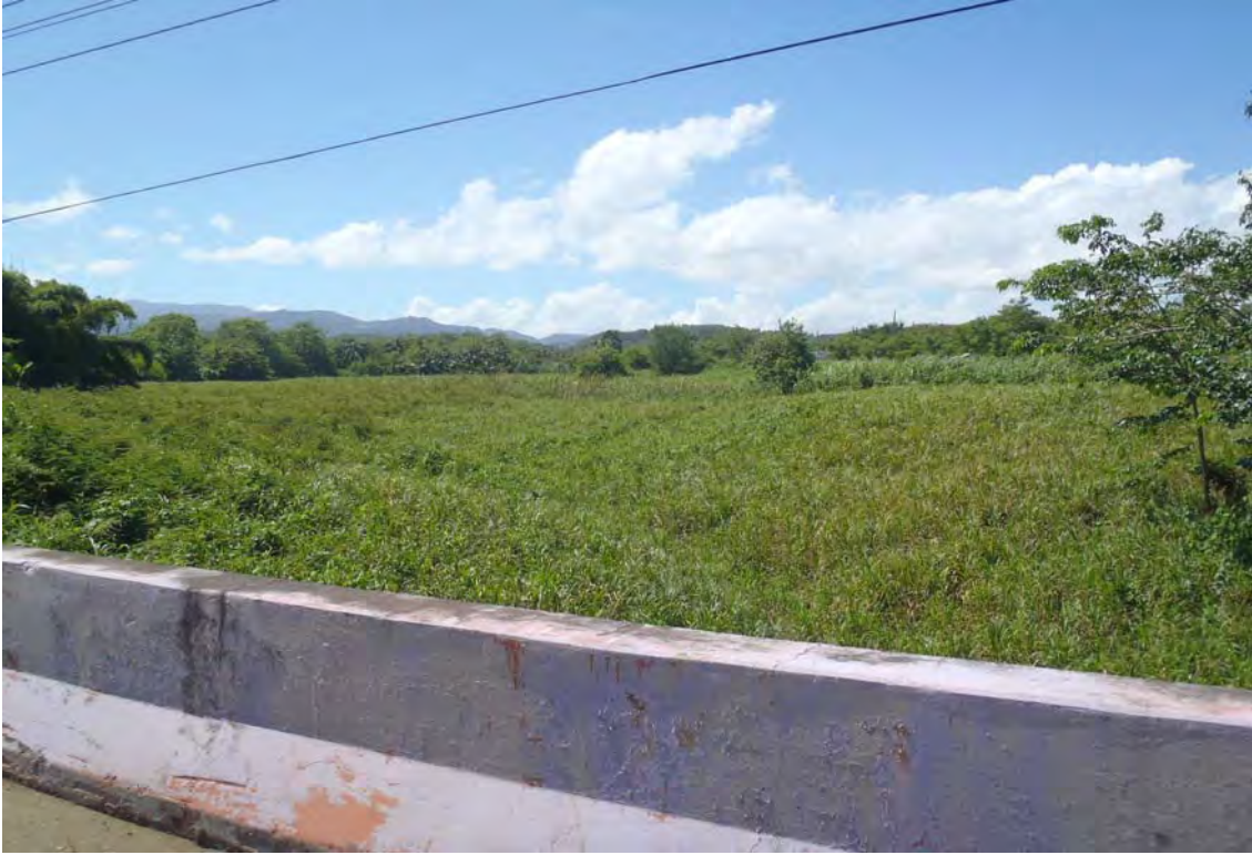
Photo 37. Point where the Quebrada Bocaforma discharges under the PR-3 towards north.
