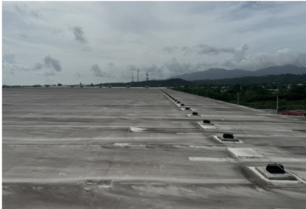
Rooftop where PV panels will be installed
