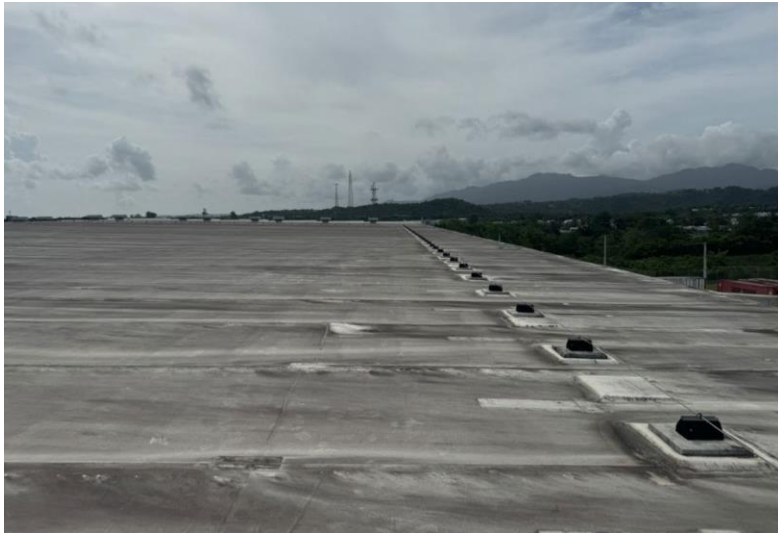
Rooftop where PV panels will be installed
