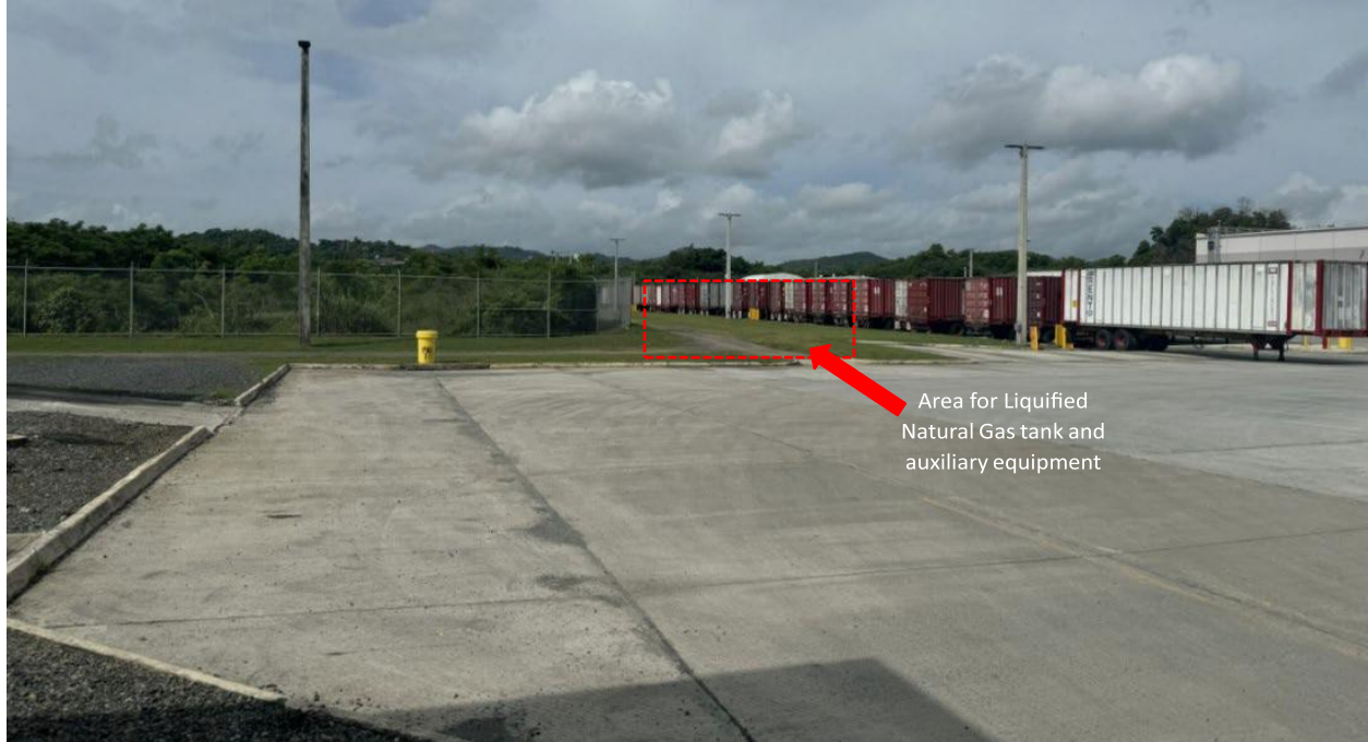
Ground-level photo showing the area where the Photo showing the area where Liquefied Natural Gas (LNG) tank and its equipment will be installed.
