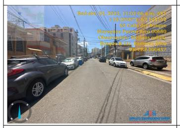
Multiple layers of asphalt create a channel between sidewalks and streets. Present in portion of Ramírez Silva Street.
