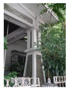
APE. Contributing and eligible property #07. Lcdo. A. Ramírez Silva Street, East view. North American California Bungalow Style. Front Porch Column Detail. © 1925-40. Materials: Reinforced concrete, masonry, wood ceilings, Creole Style floor tiles, corrugated metal panels roof finished. Photos
