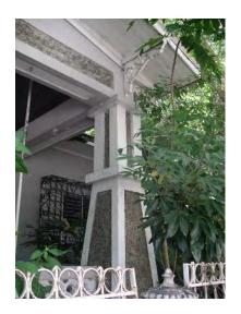
APE. Contributing and eligible property #07. Lcdo. A. Ramírez Silva Street, East view. North American California Bungalow Style. Front Porch Column Detail. © 1925-40. Materials: Reinforced concrete, masonry, wood ceilings, Creole Style floor tiles, corrugated metal panels roof finished. Photos #23-28.
