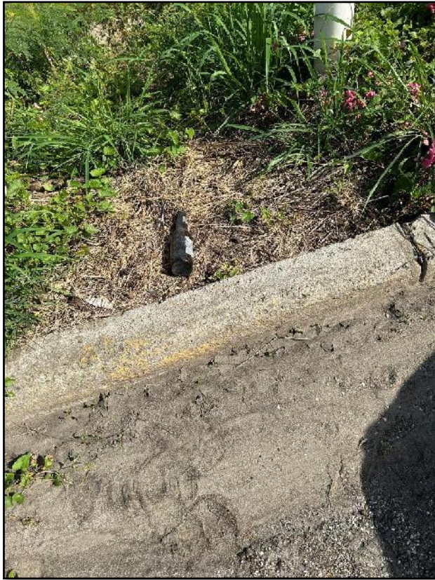
Parking Area Concrete Curb Painted with Yellow Lead Based Paint.
