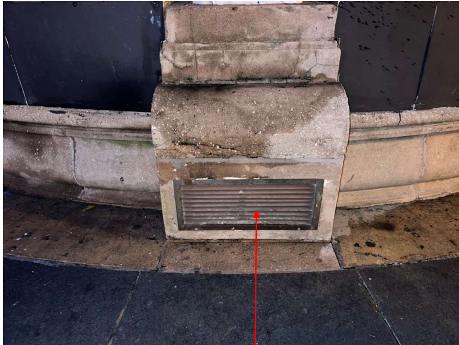
Plaza de Armas- Water Fountain- Metal Grate with Lead Based Paint
