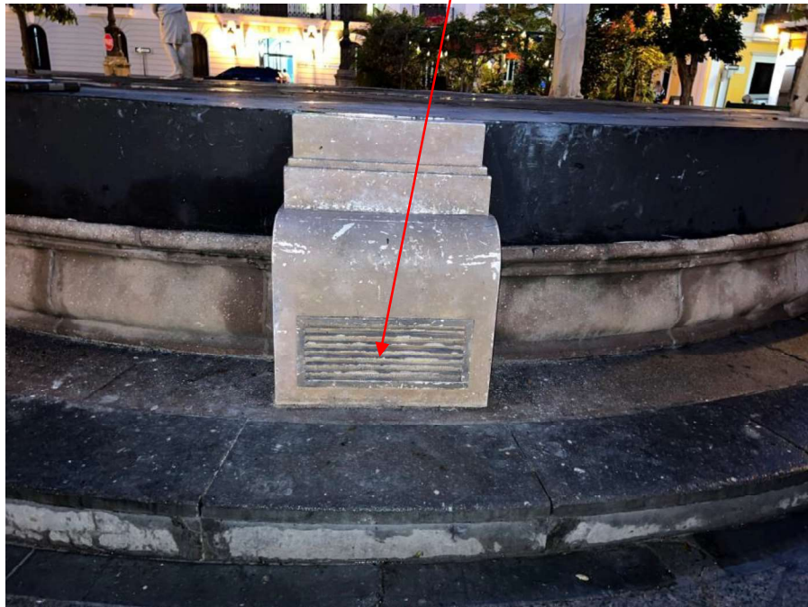
Plaza de Armas- Water Fountain- Metal Grate with Lead Based Paint
