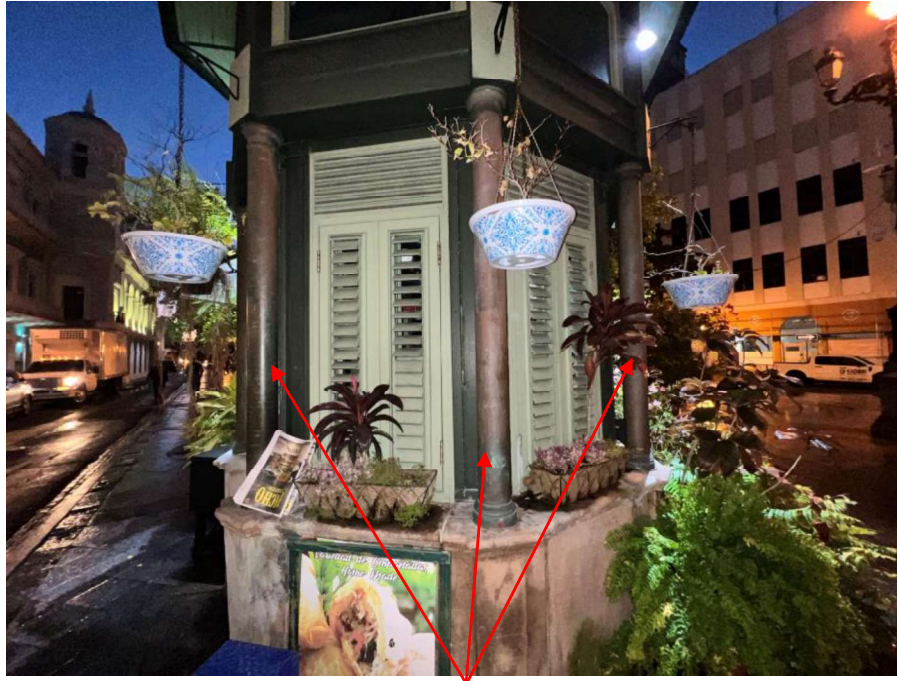
Plaza de Armas- Kiosk #1- Exterior- Metal Columns with Lead Based Paint
