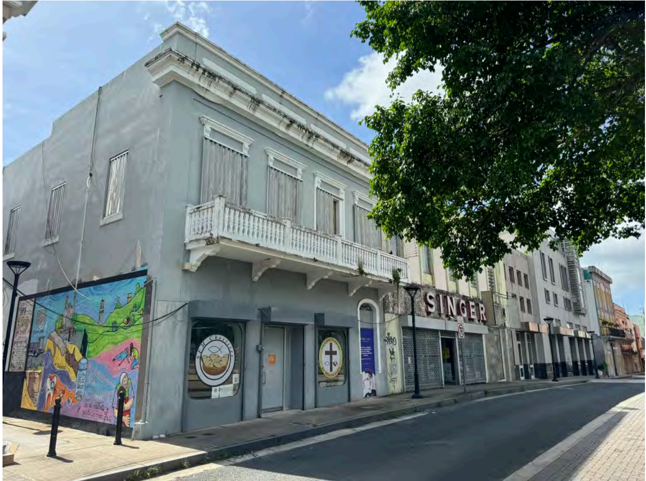
Figure 37. Early 20 th century Spanish Neoclassical commercial-residential structure built for Higinio Joglar on 1122 Ponce de Leon Avenue (Source: Author).
