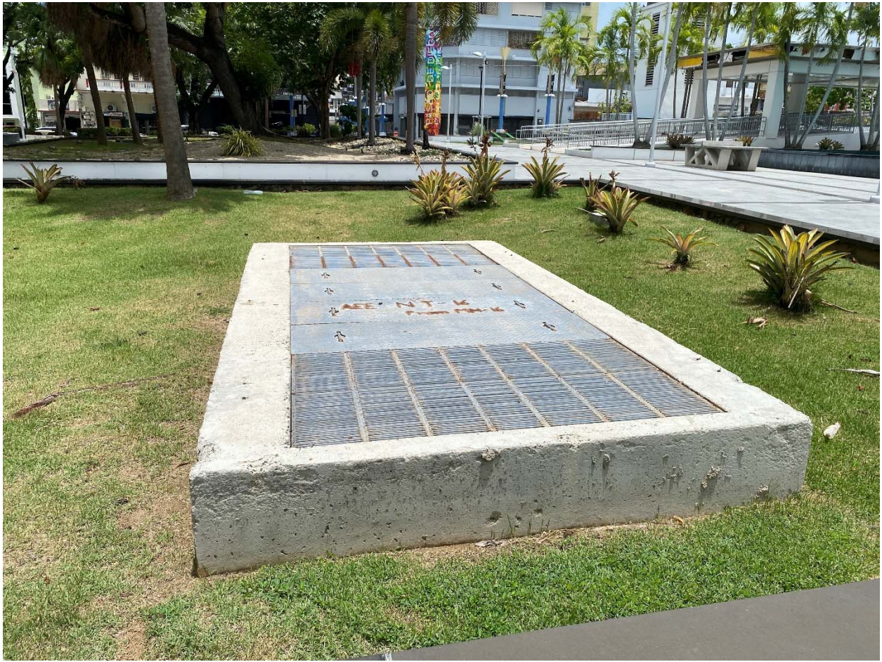
6b: Underground parking ventilation system
