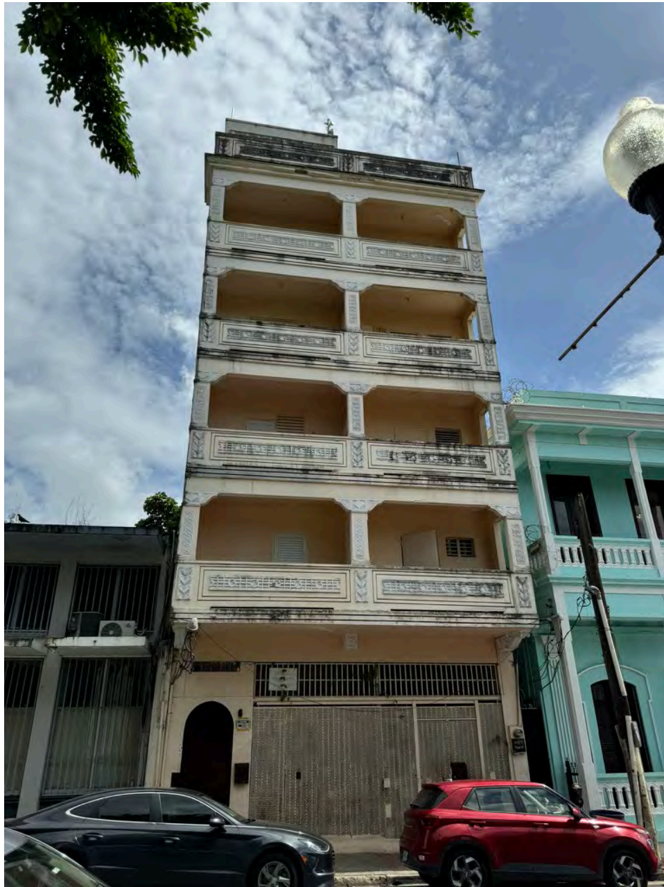
Figure 39. Dávila Monsanto Building, a 1925 Art Nouveau style five-story apartment building with retail space on the first floor on 6 Georgetti Street; the tallest building in the visual APE (Source: Author).
