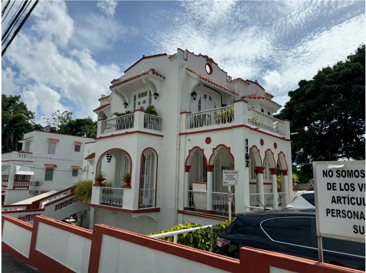
Figure 35. c. 1945 Spanish Revival residence located in 1164 Brumbaugh Street, Ubarri Neighborhood, 0.07 miles south of the APE and outside of the Visual APE (Source: Author).
