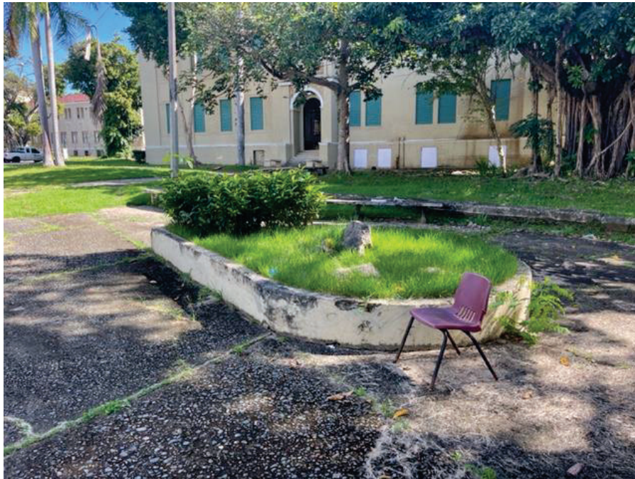
South Square Area- Concrete Planter Walls with Lead Based Paint
