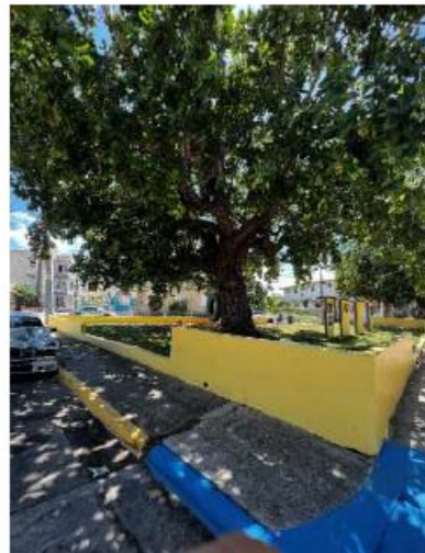
Photo 4. Detail of Raised Concrete Planter and Tree
