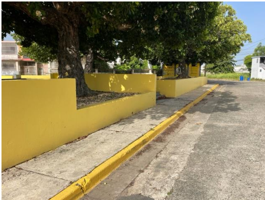
Exterior- Yellow & Blue Concrete Curbs with Lead Based Paint
