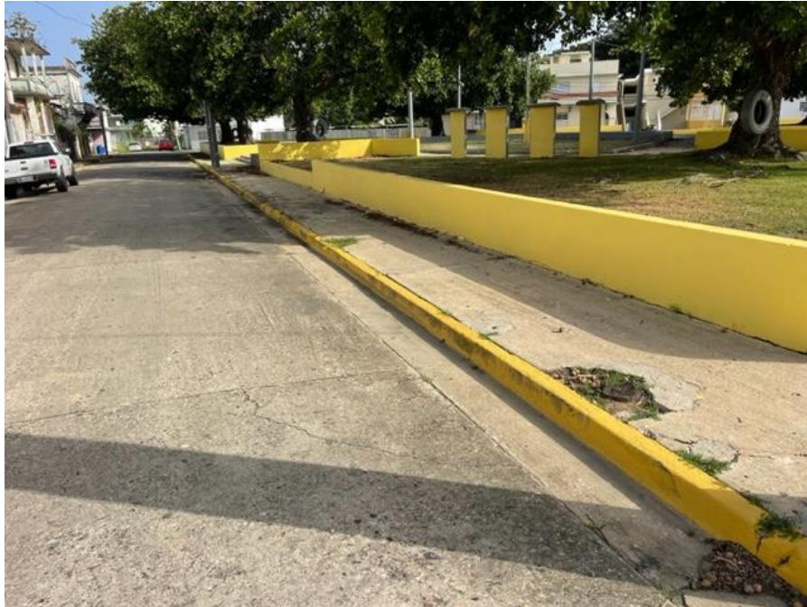
Exterior- Yellow & Blue Concrete Curbs with Lead Based Paint
