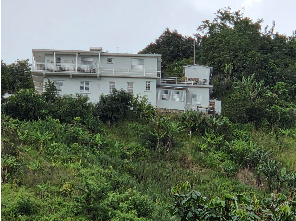
Photo 4 -.Photo showing plantain plantings established along the steep slopes where additional fruit trees will also continue to be cultivated
