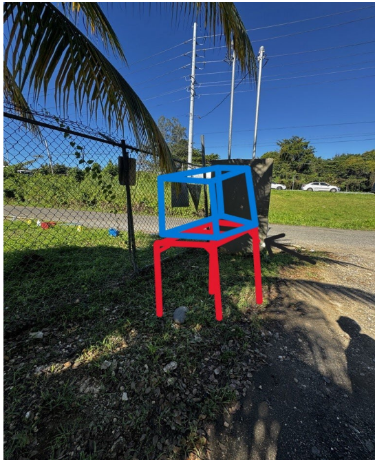
[Arrow represents transfer switch position. Red lines represent generator base. Blue lines represent the generator position. Applicant will fabricate base]
