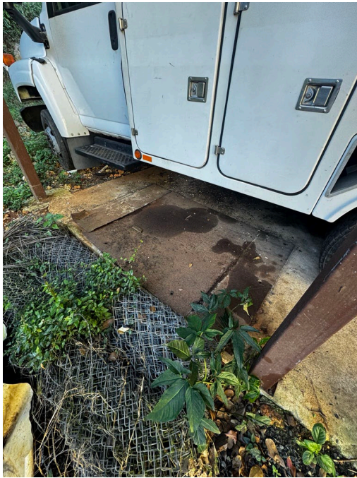
[Septic Tank Area]
