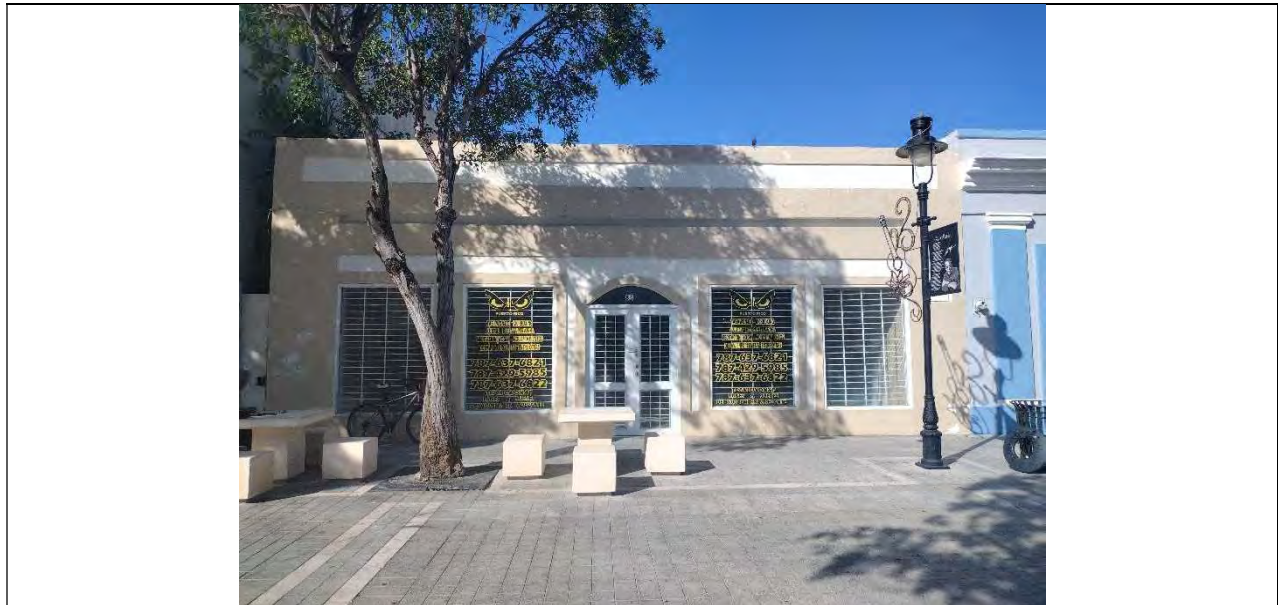
Photo #: 15 Description: Photo taken from the Paseo Atocha in Ponce (Lat. 18.01451944 Lon. -66.61394954). The photo shows the current condition of the structure. Building #85 is part of the project. Date: 11-3-2022
