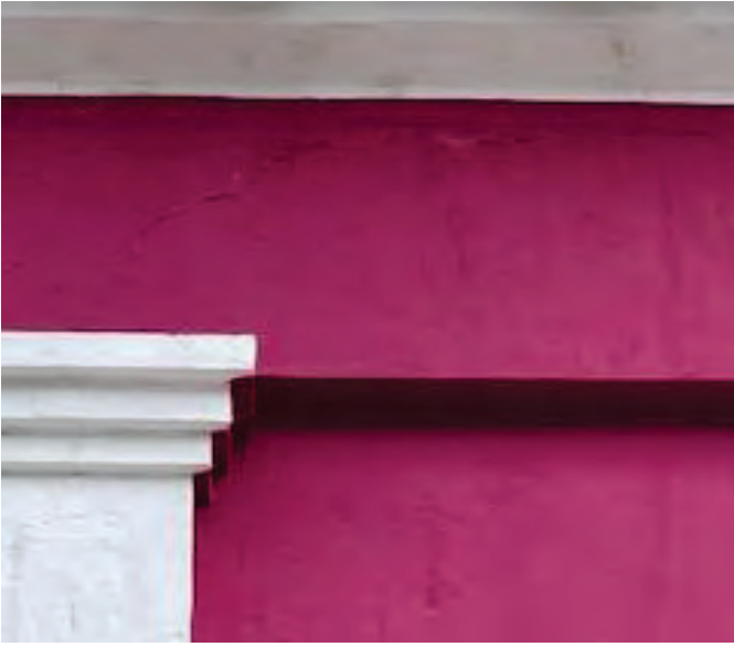
Pink/White Concrete Upper Wall/Column Painted with LBP Exterior Wall A, Building #27
