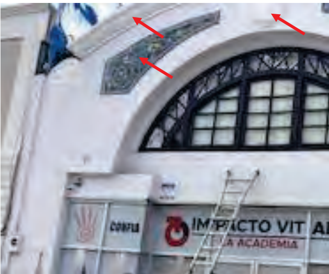
Multicolor Mosaic, White Concrete Balluster and Emblem Painted with LBP Exterior Wall A- 2nd Floor, Building #7
