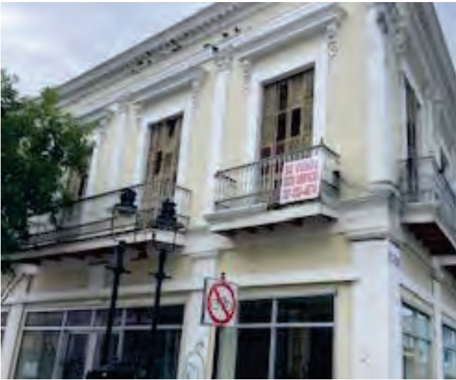
Cream Concrete Wall A, White Concrete Columns, Metal Brown Handrail White Concrete Balcony Frame and Trim, Column Decoration and Upper Trim Painted with LBP Exterior Wall A- 2nd Floor, Building #5
