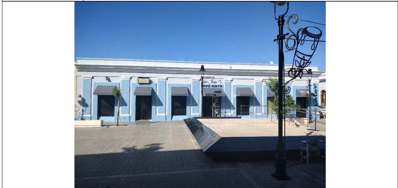
Photo #: 16 Description: Photo taken from the Paseo Atocha in Ponce (Lat. 18.01480858 Lon. -66.61404451). The photo shows the current condition of the structure. Building #87 is part of the project. Date: 11-3-2022
