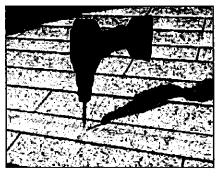
**DRILL PILOT HOLES:** Center the roof attachment over the rafter and drill a pilot hole(s) for the lag bolt(s).
