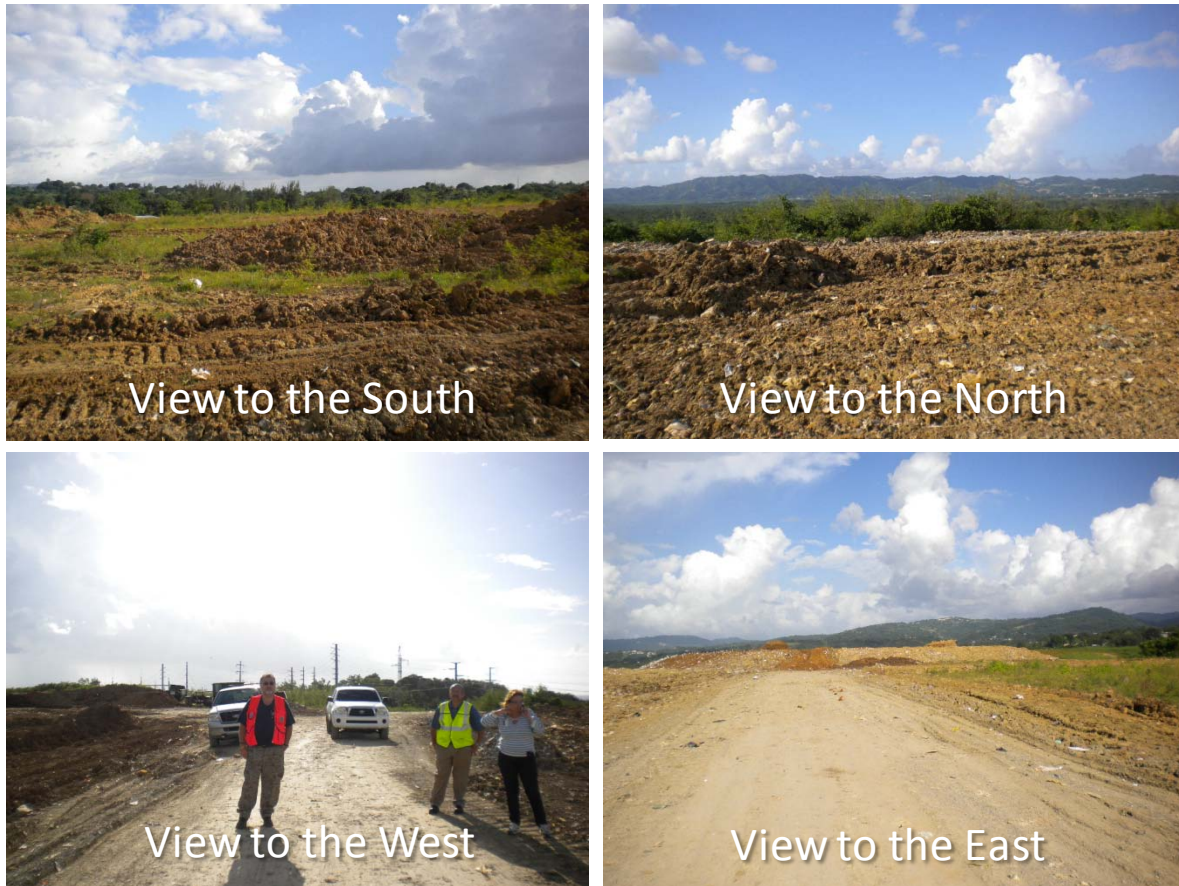
Figure 12. Views of the feasible area for PV at the Mayagüez Landfill
