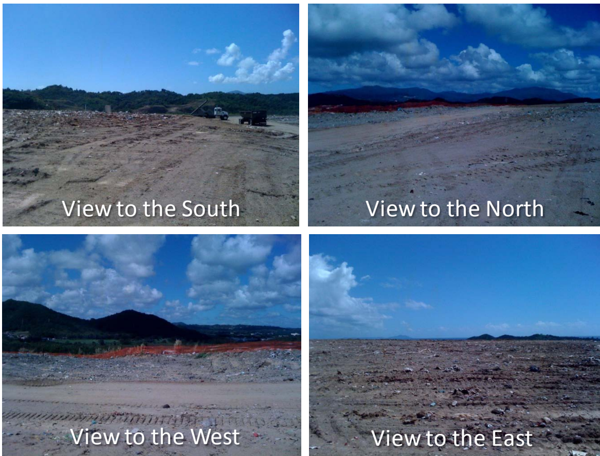
Figure 22. Views of the feasible area for PV at the Humacao Landfill
