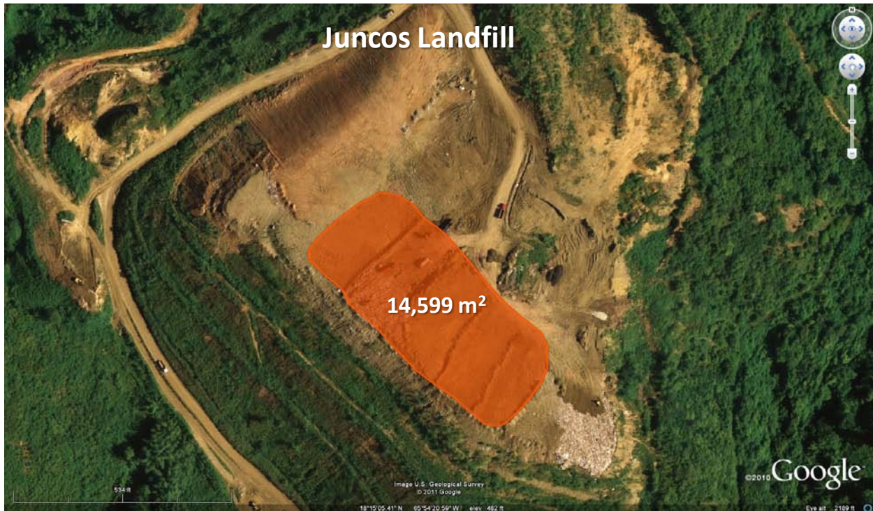
Figure 25. Aerial view of the feasible area for PV at the Juncos Landfill
