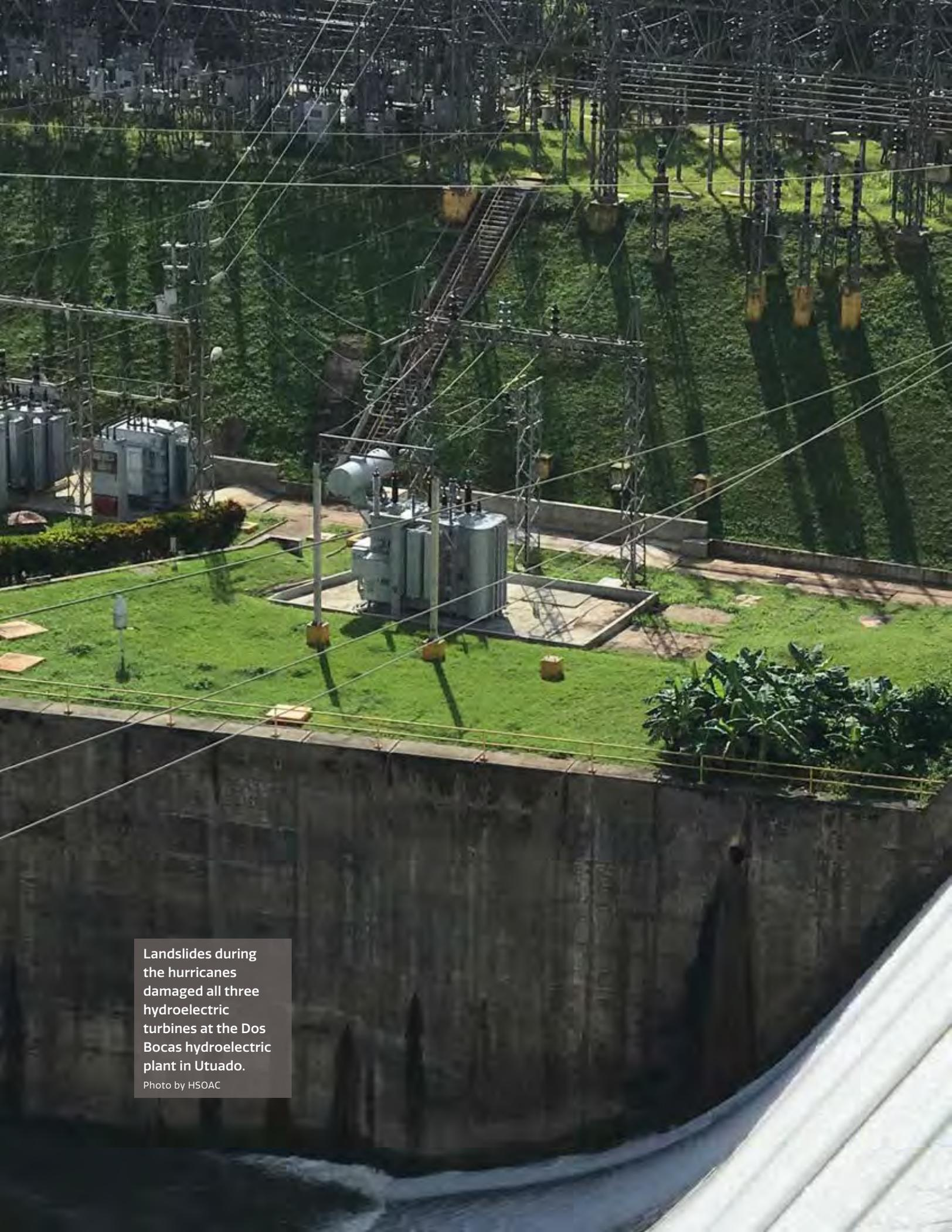
Landslides during the hurricanes damaged all three hydroelectric turbines at the Dos Bocas hydroelectric plant in Utuado.
