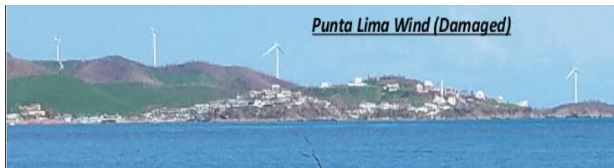
Source: NYPA/Con Edison Damage Assessments
