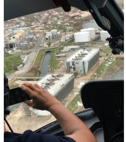
Source: NYPA/Con Edison Damage Assessments
