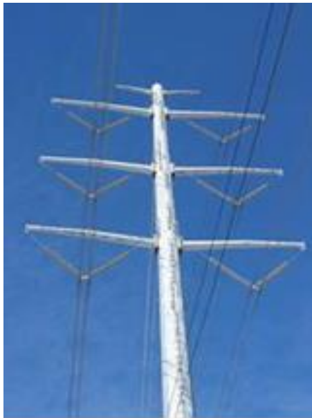
Monopole designs generally performed better than lattice tower designs.
