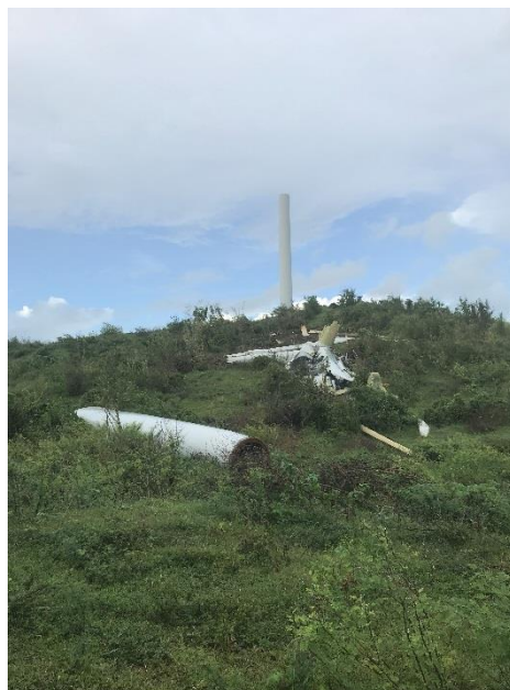
Destroyed Wind Generation
