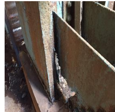
Source: NYPA/Con Edison Damage Assessments
