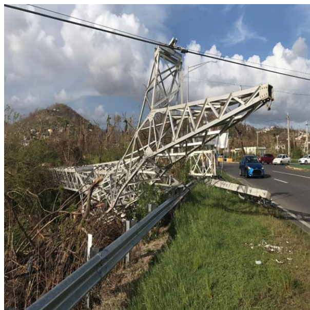
Monopole designs generally performed better than lattice tower designs.
