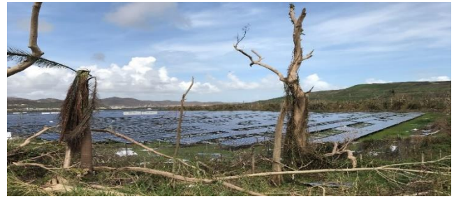
Source: NYPA/Con Edison Damage Assessments
