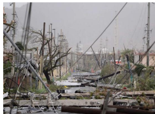
Source: NYPA/Con Edison Damage Assessments
