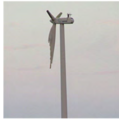
FIGURE 2. A damaged wind turbine with two of its blades broken at their neck and the third blade delaminated. (Photo: A. Kwasinski).
