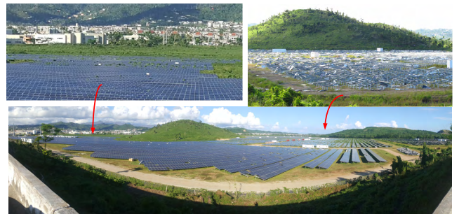
FIGURE 3. The PV "farm" at Humacao. The bottom image, facing north, shows a general view of this facility. A hill at the center of this image may have protected the central area of this facility. A detail on the top and right of this general view shows the nearly completed expanded area from the eastern side, facing west, towards the central hill. The detail on the top left shows damage west of the hill as seen looking from the south of the facility. (Photo: A. Kwasinski).
