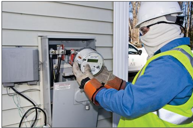
Figure 6-5. Example of AMI Meter Training
