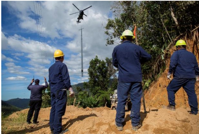
Figure 2. PREPA Rebuild Aerial Operation
