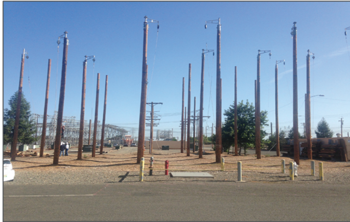
Figure 6-4. Training Yard with Facilities (T/D Overhead and Underground)
