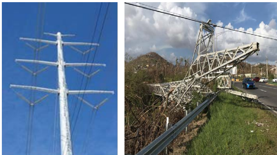
Figure 4-5. Monopole vs. Lattice Tower Design
