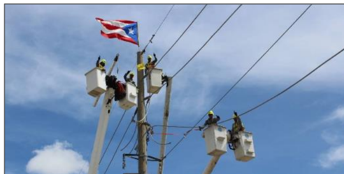
Figure 4-7. Distribution Line Repairs
