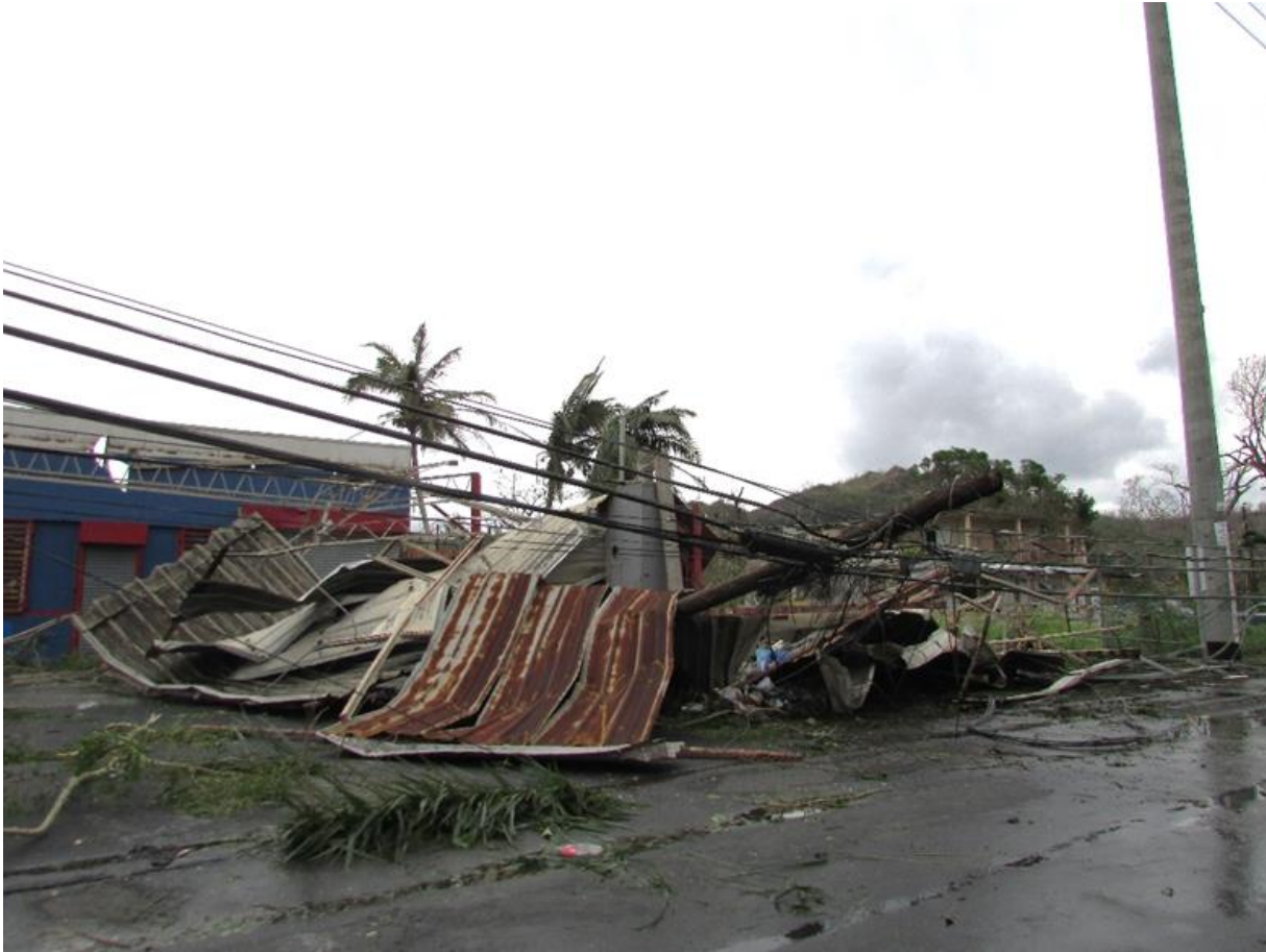
Figure 26 - Wooden electrical distribution pole damaged by Hurricane María at Trujillo Alto, Puerto Rico
