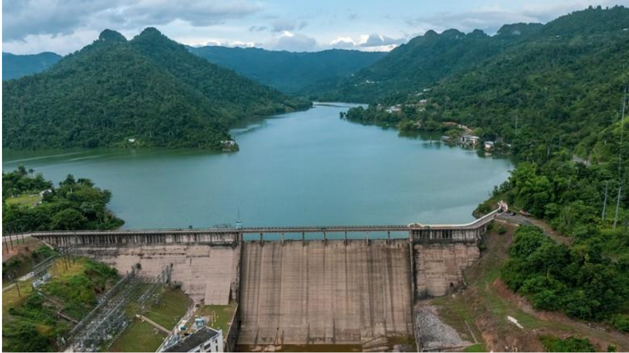
Figure 2 - Dos Bocas Hydroelectric Plant
