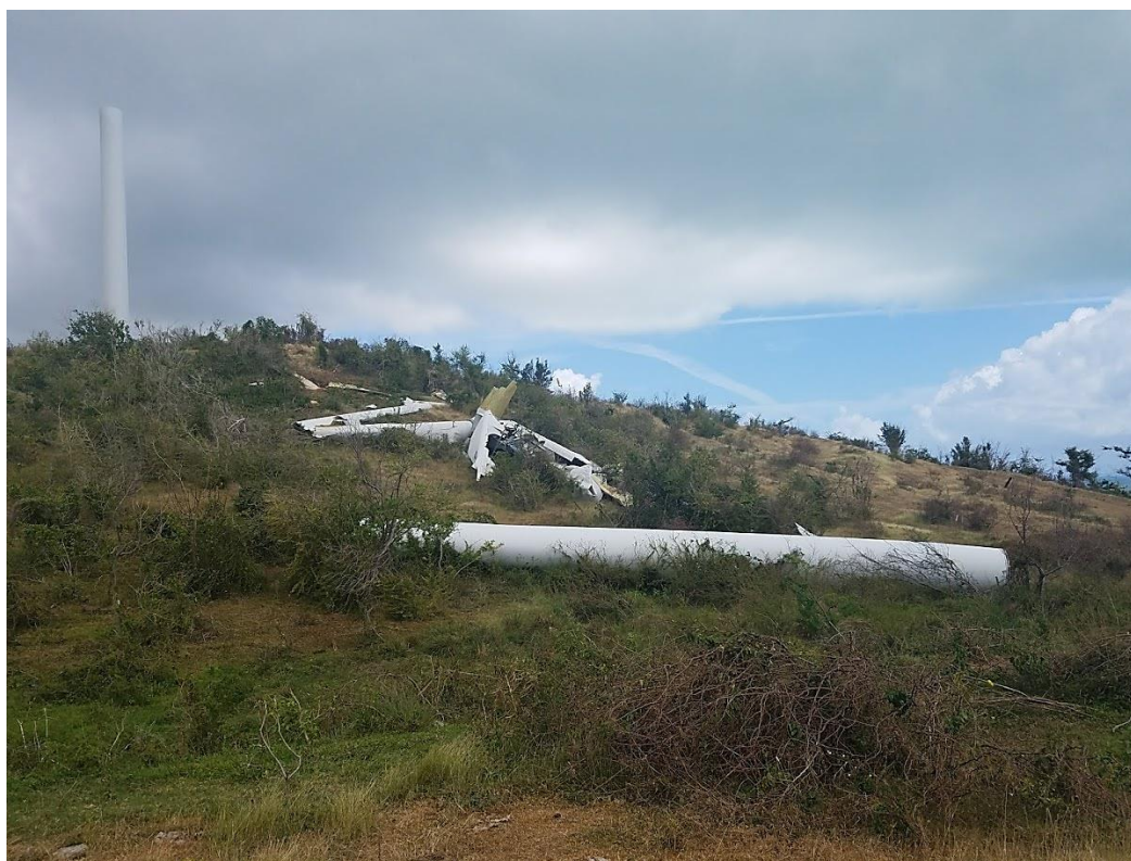
Figure 25 - Inoperable and damaged wind turbines at Punta Lima wind farm after Hurricane María in Naguabo, Puerto Rico
