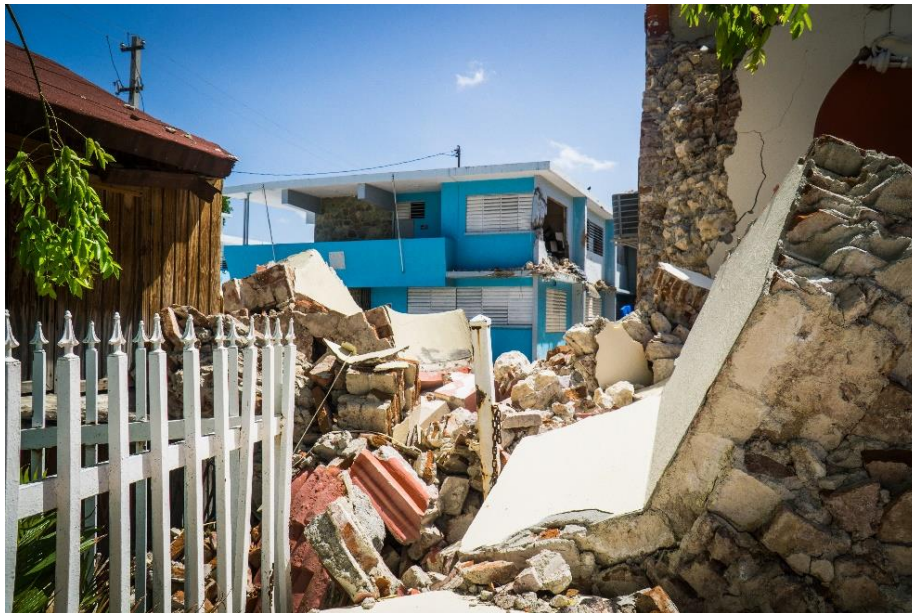
Figure 2: Damage from 6.4 earthquake on January 7, 2020 in Guayanilla
