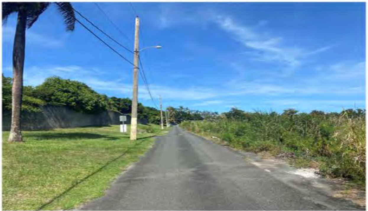
PHOTO 5- VIEW OF SECTOR SARDINERA ROAD (WESTERN BOUNDARY) TOWARDS NORTH
