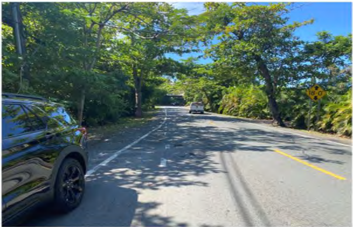
PHOTO 6- VIEW OF STATE ROAD PR-693 (SOUTHERN BOUNDARY) TOWARDS WEST
