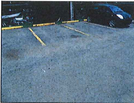
Exterior Parking Area Lead based painted parking pavement marking
