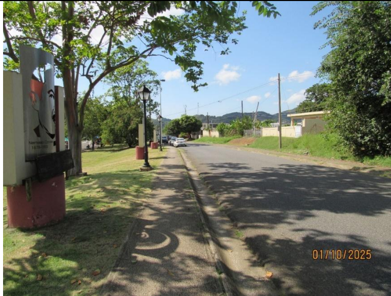
Photo #17 Looking Southwest from La Colonia Ave. toward the project 01/10/2025 18.004738, -66.008821
