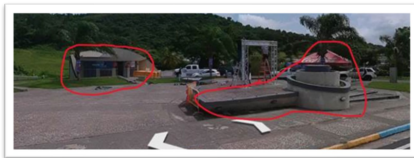
Figure 5 – Image with Existing restroom building (left) and platform to be demolished (right)
