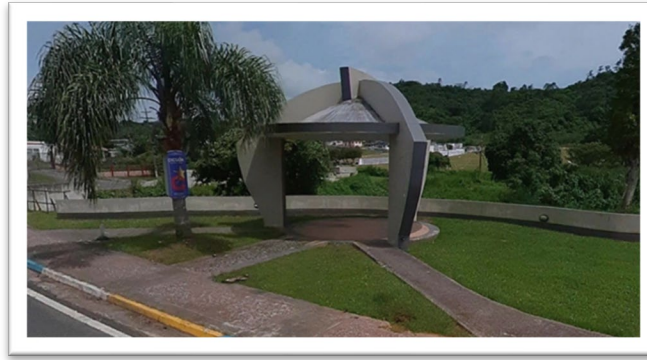
Figure 4 – Front view of Existing Gazebo at Las Flores Bike Trail Plaza
