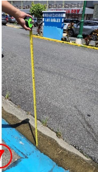
Photo location # 8- Existing sidewalks showing no ADA compliance width.
