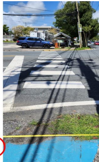
Photo location # 2- Existing sidewalks showing no ADA compliance width.
