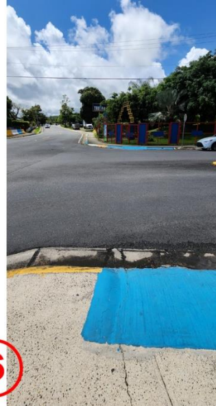
Photo location # 7- Existing cross walk whit no ADA compliance ramp.
