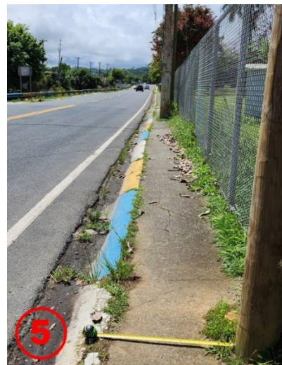
Photo location # 5- Existing sidewalks showing no ADA compliance width.
