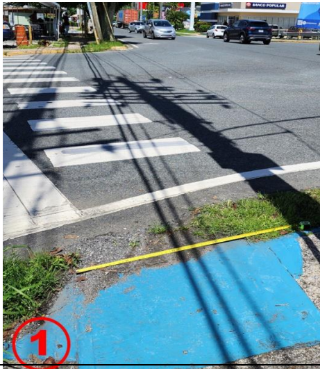
Photo location # 1- Existing sidewalks showing accessibility barriers- ramps non-ADA compliance.
