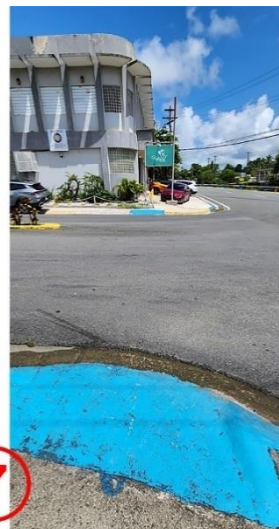
Photo location # 7- Existing cross walk whit no ADA compliance ramp.
