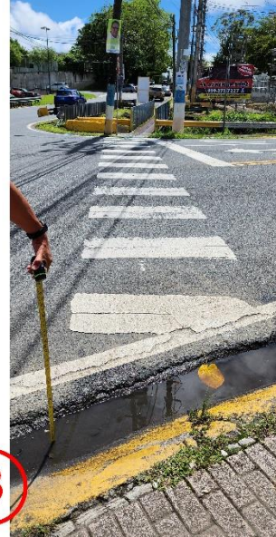
Photo location # 5- Existing sidewalks showing no ADA compliance width.
