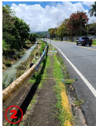
Photo location # 2- Existing sidewalks showing no ADA compliance width.
