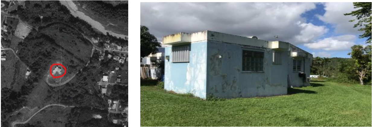
Figure 1 & 2. Detail of 1994 aerial image showing the building on the property, and the rear elevation, view to the northwest.
