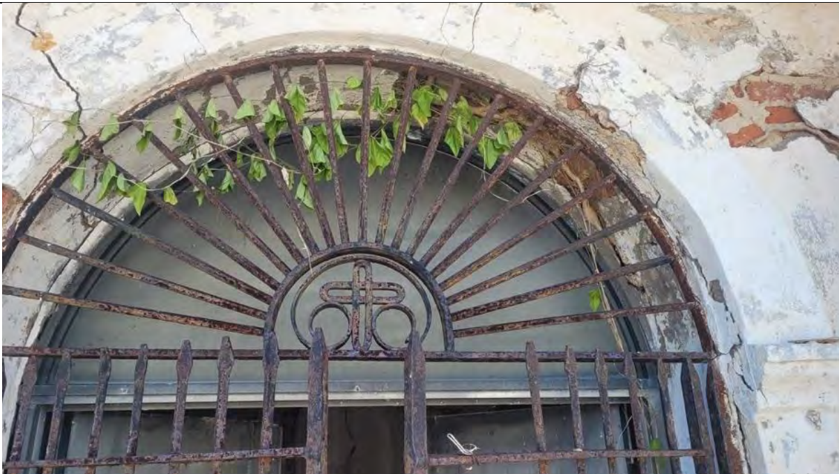
40.2 Entrance arch to the mausoleum. Bricks in walls are visible along with deteriorated metal gates.
