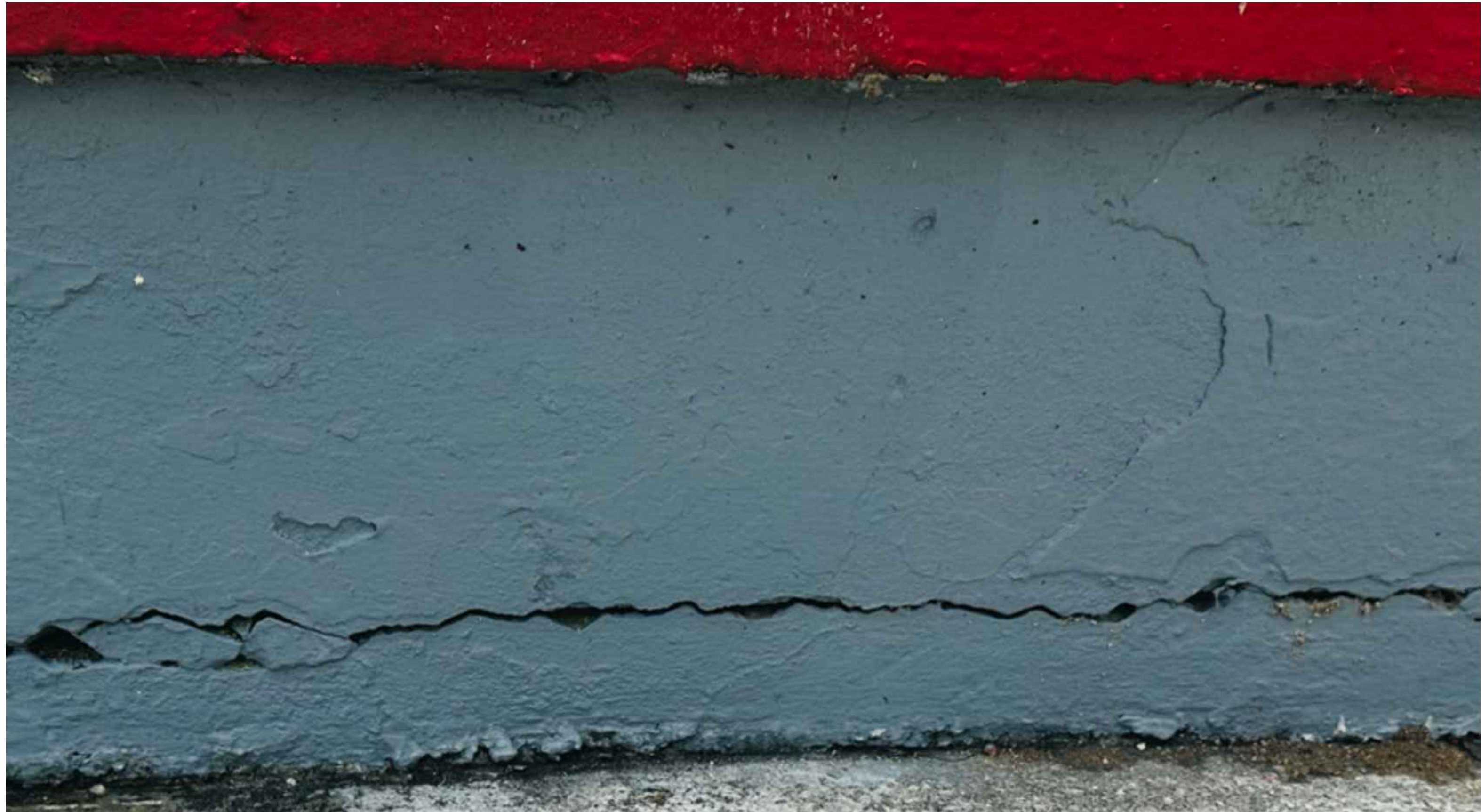
PH-9 Existing conditions of the plaza (broken concrete and deterioration)
