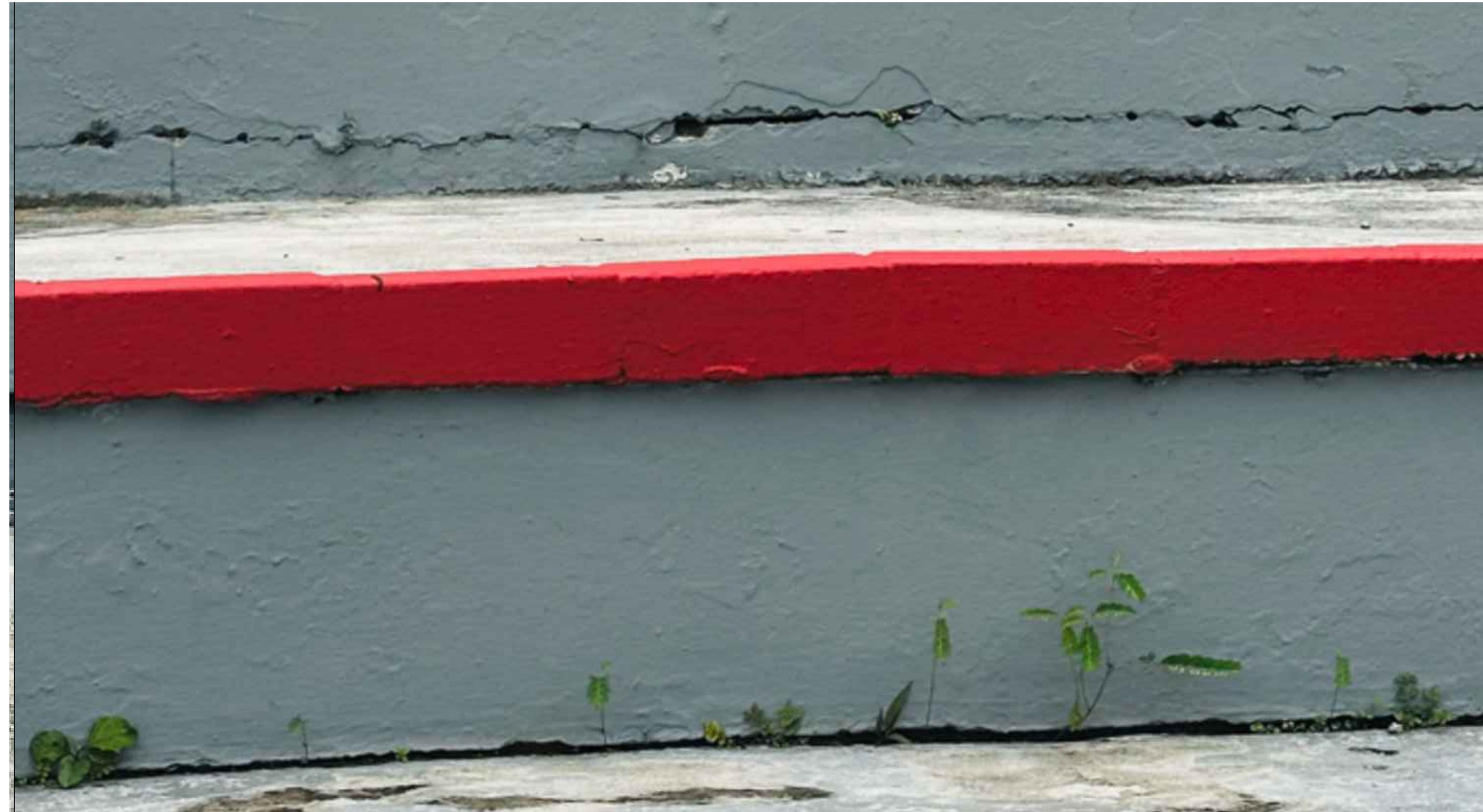
PH-11 Existing conditions of the plaza (broken concrete and deterioration)
