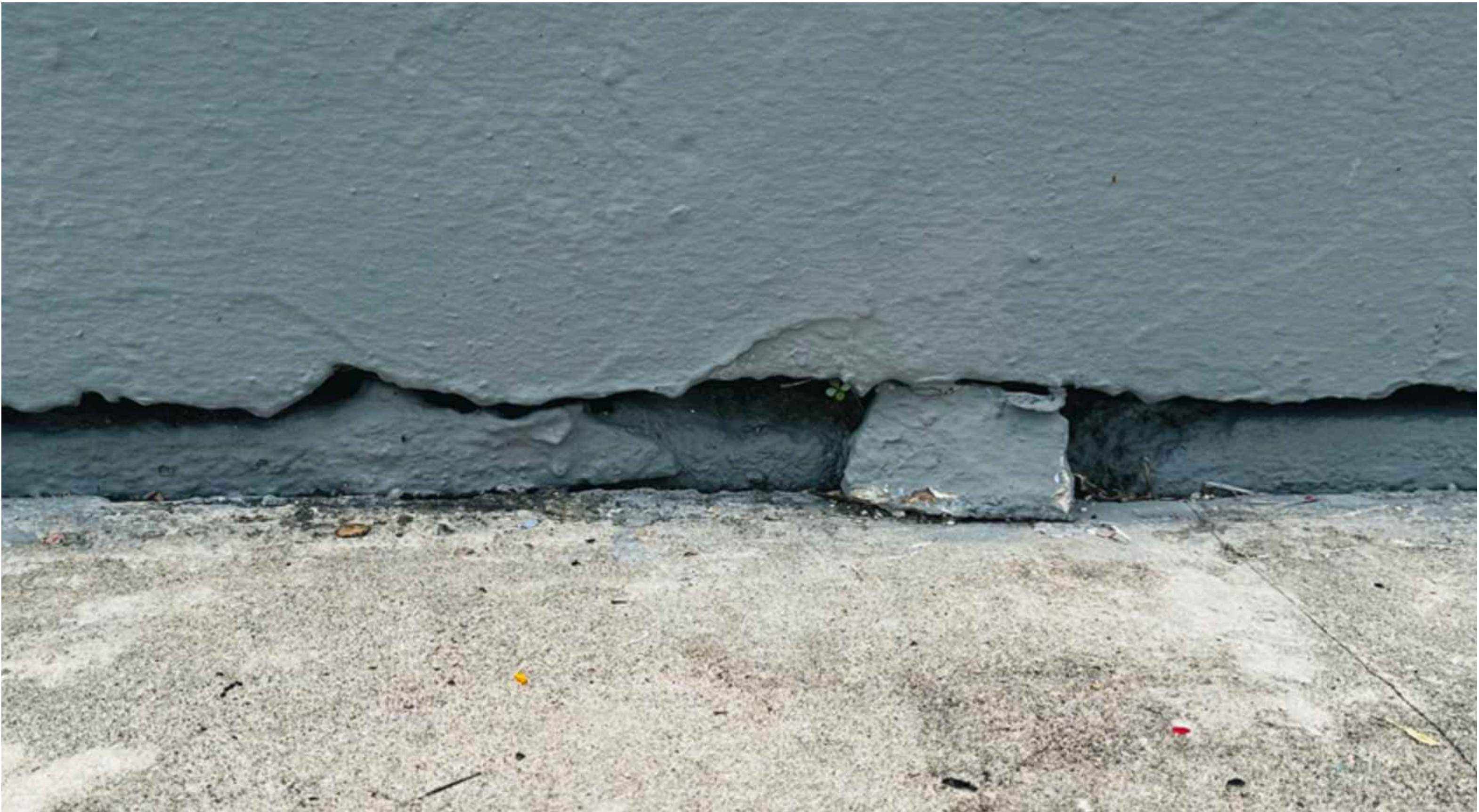
PH-10 Existing conditions of the plaza (broken concrete and deterioration)
