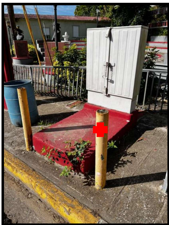
Figure 6: Electrical Cabinet (Yellow bollards tested positive)
