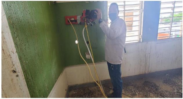
Photo 4: Core specimen were extracted from walls selected by Structural Consultant.
