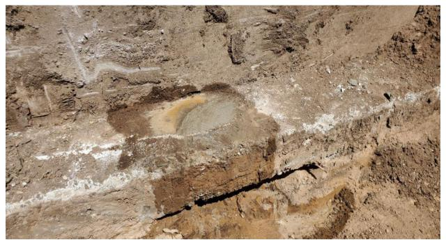
Photo 17: Core specimen extracted from footing were backfilled with high strength mortar.
