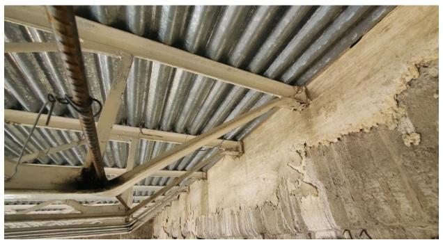
Photo 21: Steel joist are embedded in the concrete wall/
