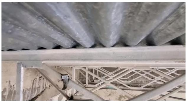
Photo 23: Connection between steel joist or metal deck with slab were not found.
