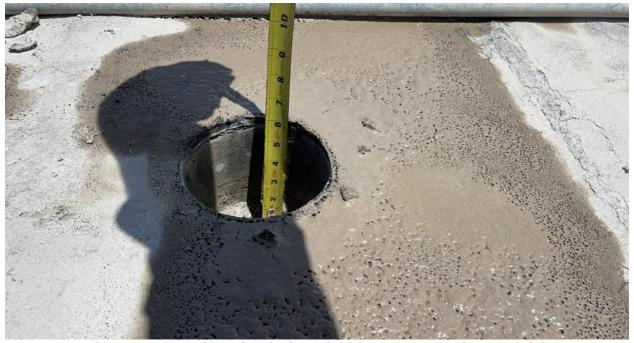
Photo 10: Approximately 6 inches of thickness measured on roof slab.
