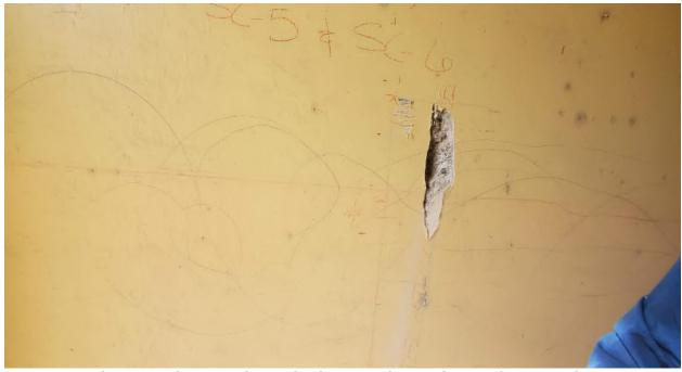
Photo 2: Rebar were located using scanning equipment for extraction.
