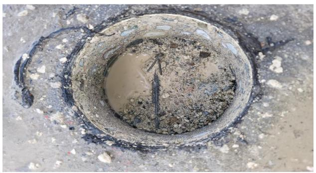
Photo 11: Connection between roof slab and metal deck or steel joist could not be found.
