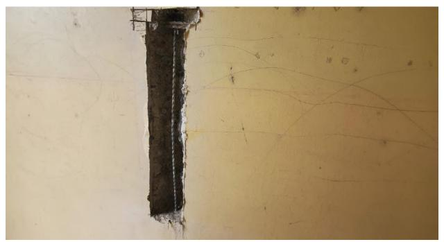
Photo 3: Rebar was exposed on at least 36 inches to be extracted for laboratory testing.
