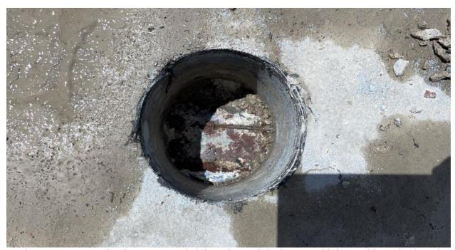
Photo 14: Connection between roof slab and metal deck or steel joist could not be found.
