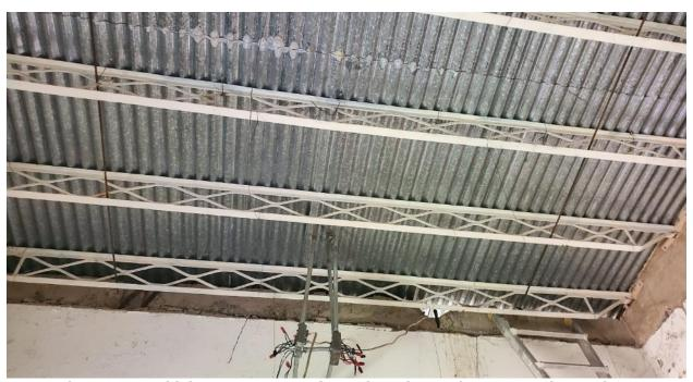
Photo 18: Steel joist were measured on selected areas by Structural Consultant.
