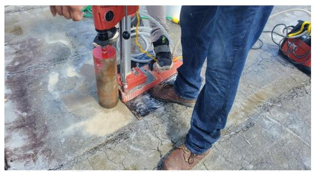
Photo 6: Core drills were performed on roof slab selected by Structural Consultant.
