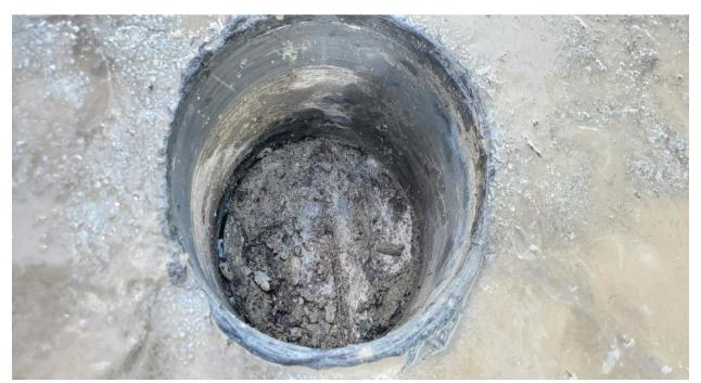
Photo 9: Roof slab was not connected with exiting metal deck or steel joist below.
