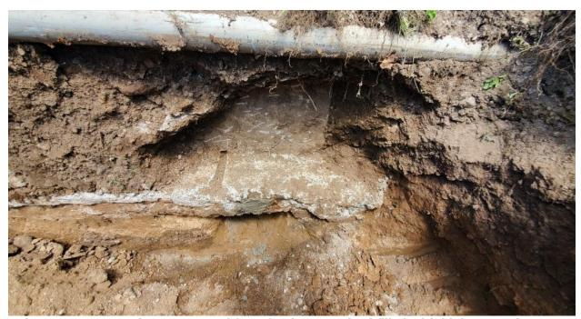
Photo 16: Core specimen extracted from footing were backfilled with high strength mortar.
