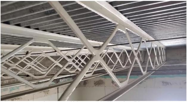
Photo 20: Steel joist were noticed in good conditions.
