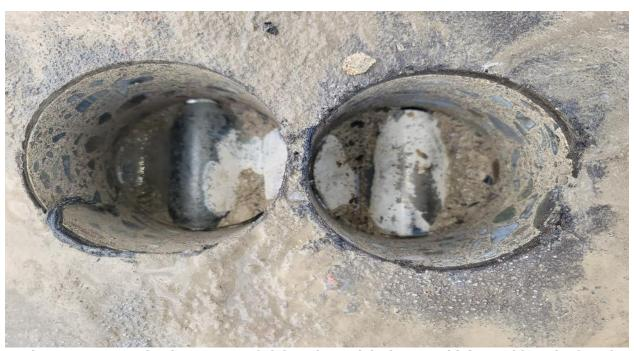
Photo 12: Connection between roof slab and metal deck or steel joist could not be found.
