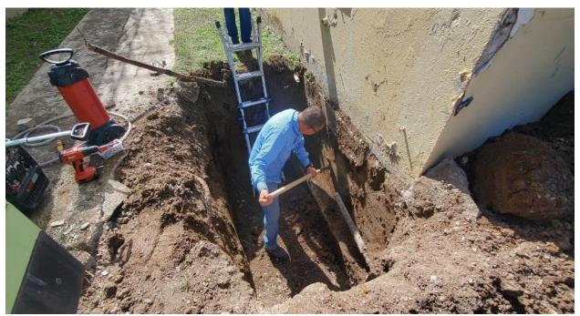
Photo 15: Footing dimensions were taken on excavation areas.
