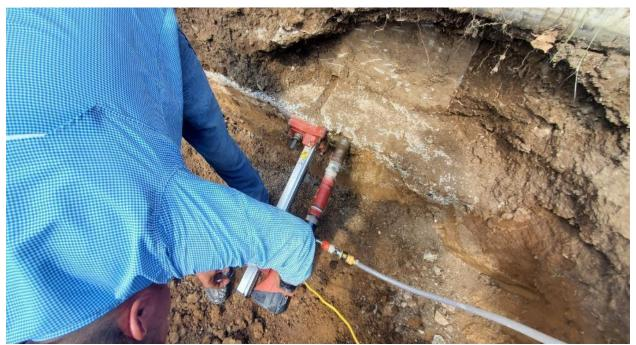
Photo 5: Core specimen were extracted from footings selected by Structural Consultant.
