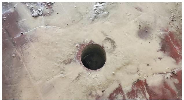
Photo 7: Core drills were performed on second level slab selected by Structural Consultant.
