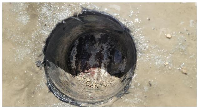
Photo 13: Connection between roof slab and metal deck or steel joist could not be found.
