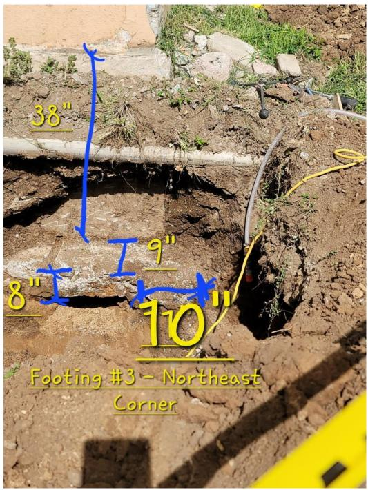
Photo 59: Footing #3 measurements on norhteast side excavation.
