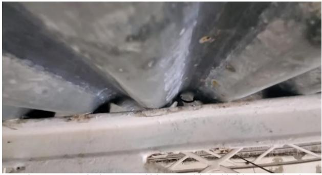
Photo 22: Connection between steel joist or metal deck with slab were not found.
