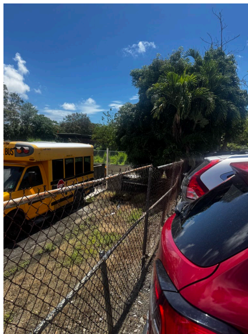
Chain link fence to be repair
