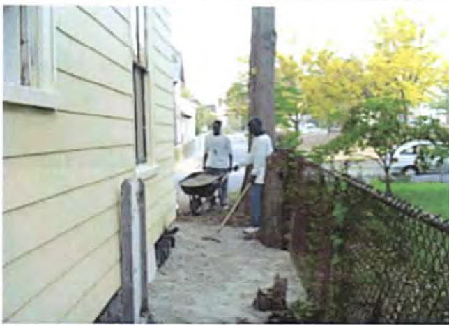
FIGURE 12.23 Preparing to pave high traffic area.
