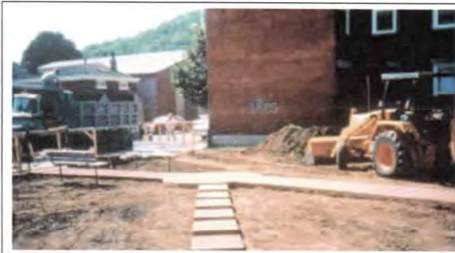
FIGURE 12.22 Replacing resident pathway after soil removal.
