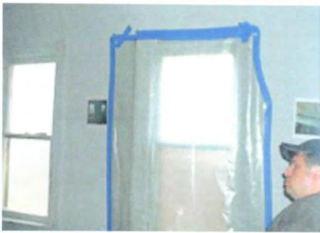
FIGURE 12.2 Protecting the interior of a unit for exterior window abatement.
