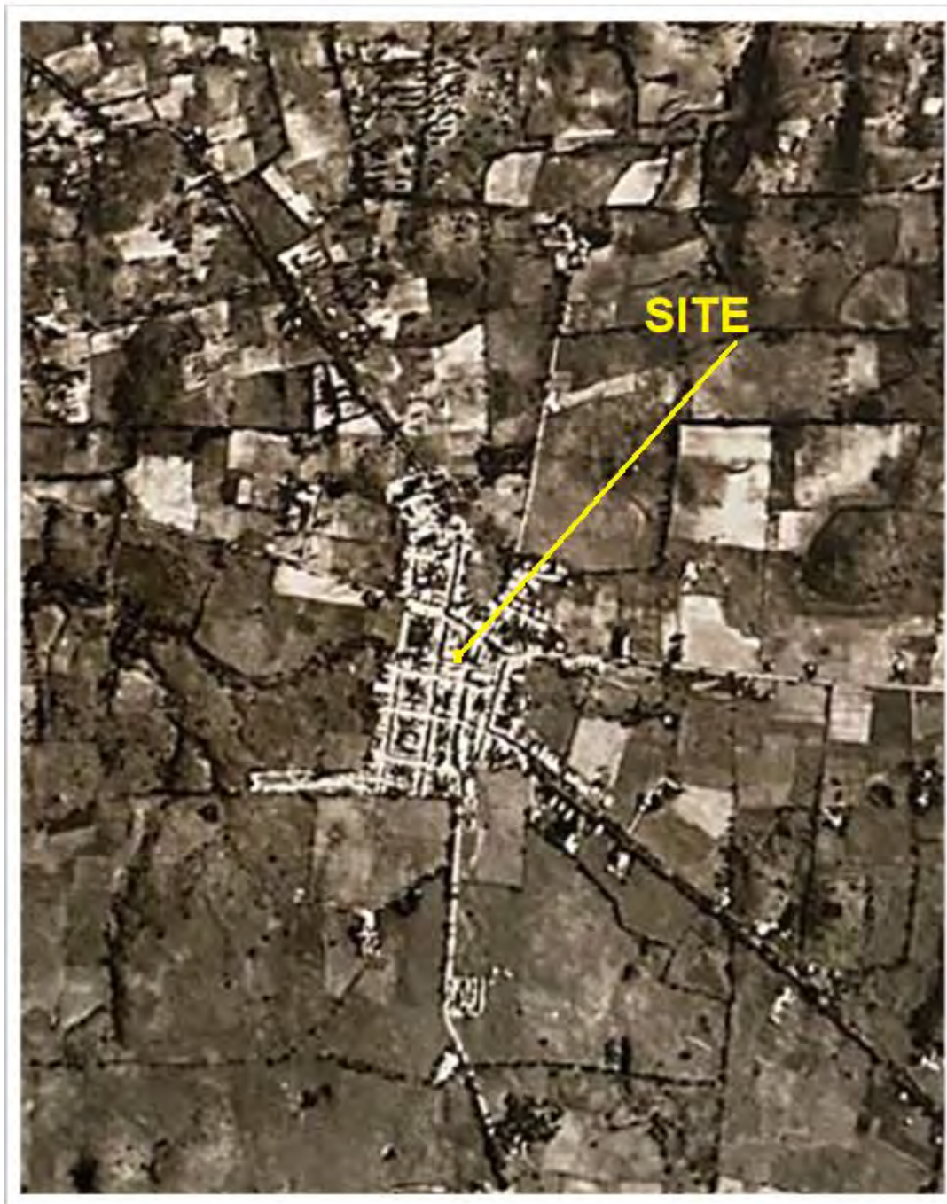
Figure 4: Quebradillas Urban Center in 1936. Aerial photo, DTOP.
