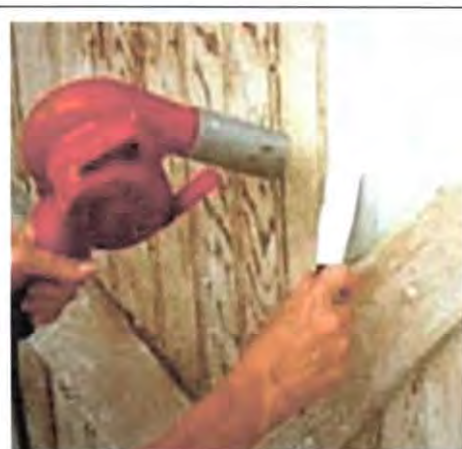
FIGURE 12.14 Using a heat gun to remove paint is labor-intensive.
