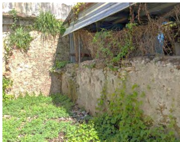
Figure 4: Bricks and mortar masonry wall at the posterior courtyard (from Alvarado and Ferrán 2023)
