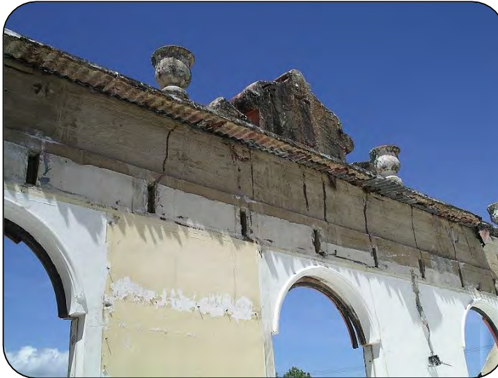
Photo: #09 Description: Second floor level interior. South view and main façade posterior concrete wall with arched doors fenestrations. Coat of arms at center of parapet with urns. Date: 07/22/22
