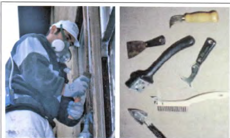
FIGURE 12.16 Wet scraping (left)
