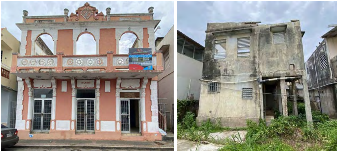
Figure 3: Frontal façade (left) and posterior façade (right) (Ingenieros del Oeste C.S.P 2022)
