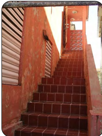
Photo: #02 Description: South-East view. Stairs on side courtyard to second floor. Date: 07/22/22
