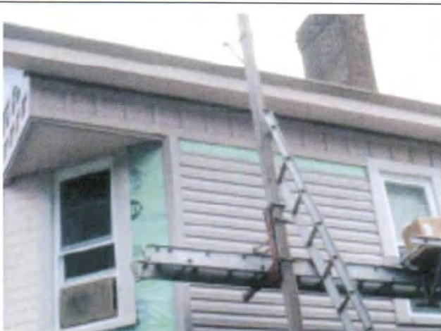
FIGURE 12.6 Installation of replacement siding.
