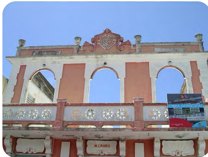
Photo: #10 Description: South view of second floor level main façade. Concrete wall with arched doors fenestrations and decorative elements on wall surface and balcony Date: 07/22/22
