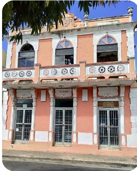
Photo: #01 Description: South view and main façade located at Honorario Hernández Street Date: 07/22/22
