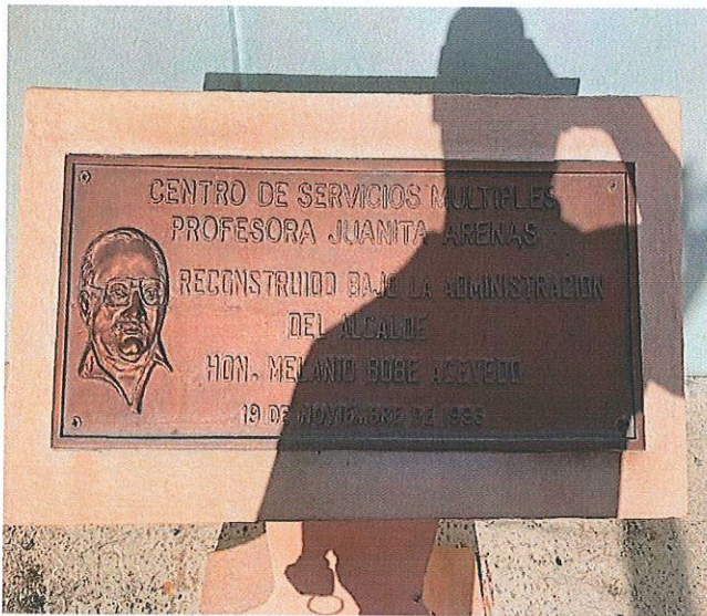
Brown Metal Commemorative Plaque Painted with LBP Exterior of Structure
