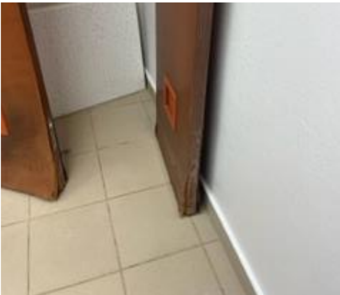
General Condition of VIP Room- Bathroom Wood Doors with Visible Water Damage
