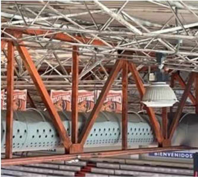
Visible Mold on Metal Joist on Ceiling
