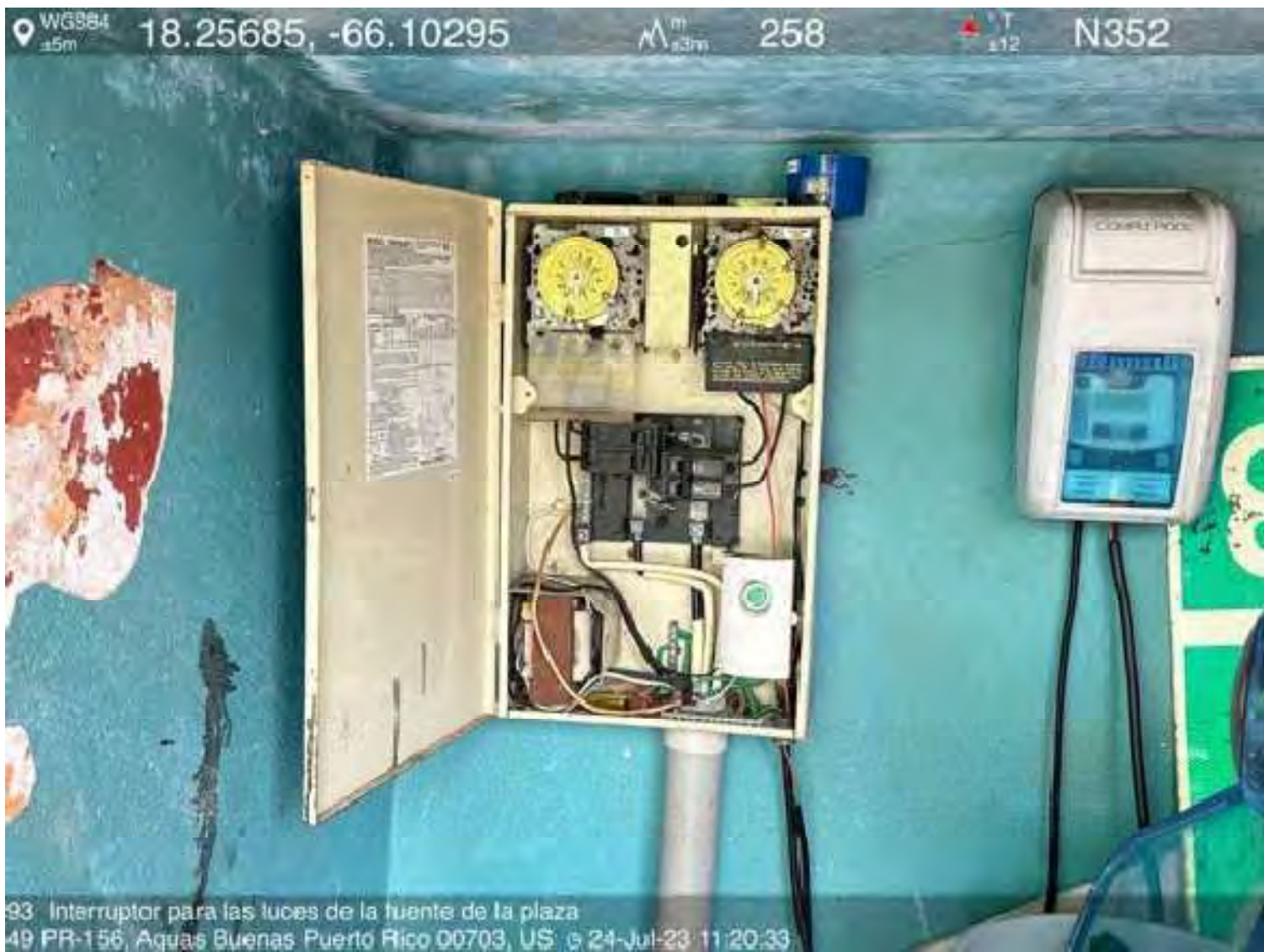
2 EXISTING SWITCH - FOUNTAIN LUMINAIRE SCALE: NOT TO SCALE
