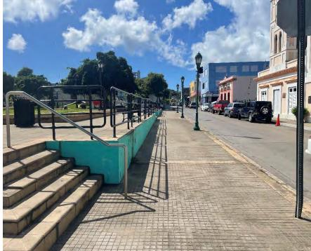
Figure 23 View of the Carlos Lebrum street and plaza (at the left of the photo). The unevenness in the slab is visible compare with the previous photo showing what was filled.
