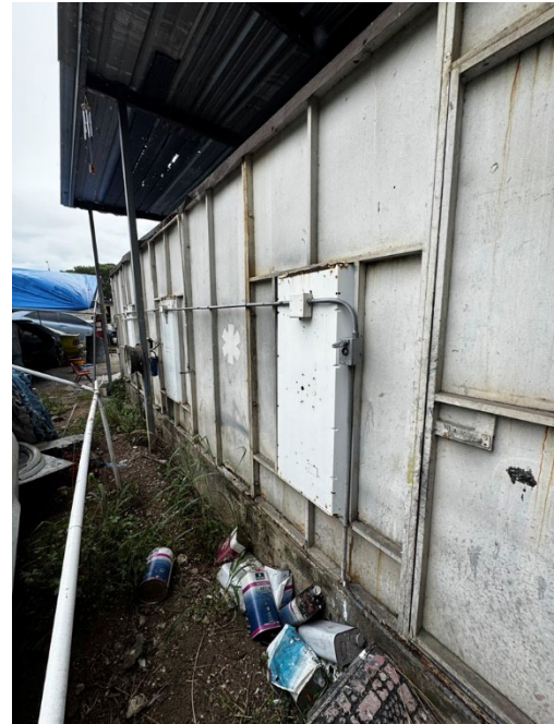
Connections at the 3 rd Structure
