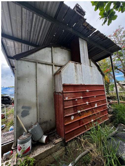
Rear of the Property 3 rd Structure
