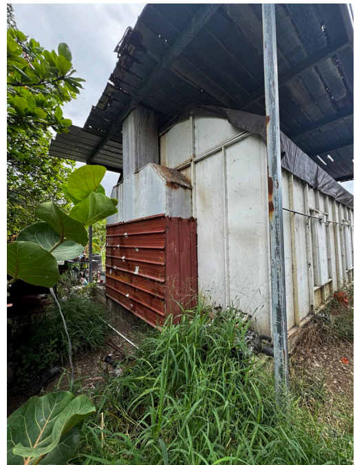
Rear of the Property 3 rd Structure
