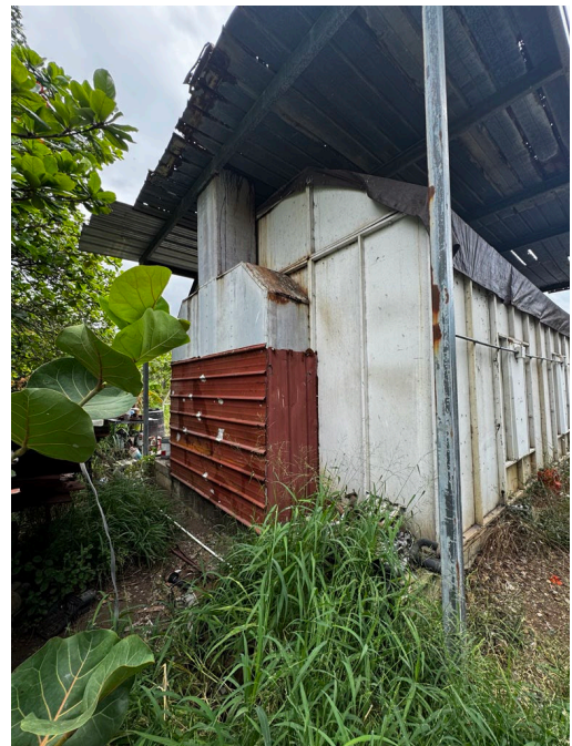
Rear of the Property 3 rd Structure
