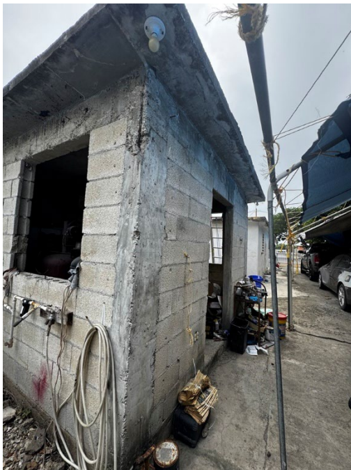
Left Side of the Property 2 nd Structure
