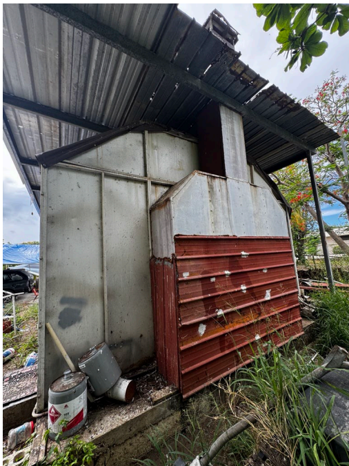
Rear of the Property 3 rd Structure
