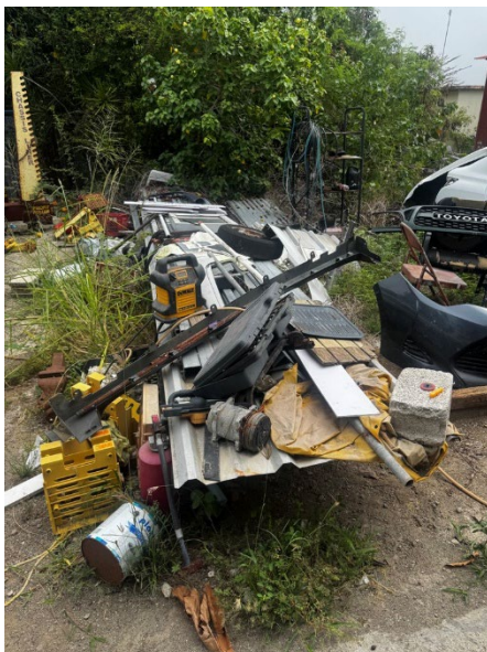
Pile of materials to rebuild roof affected
