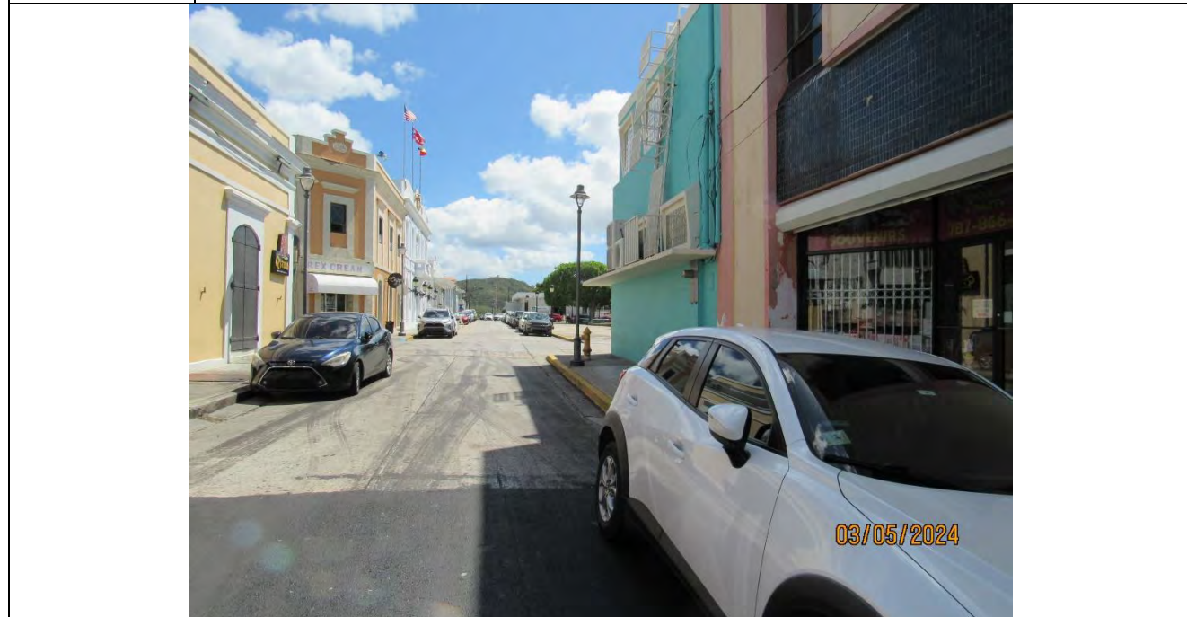
Photo #20 3/5/2024 View from Pales Matos Street (17.985666, -66.114257) looking East towards the Plaza
