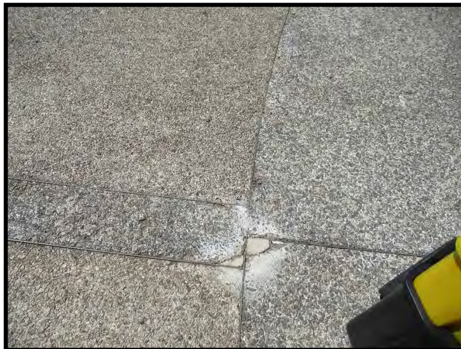
Figure #3: Floor concrete slab (PPG-02)
