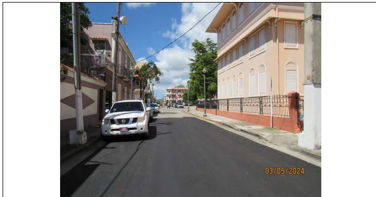
Photo #7 3/5/2024 View from Derkes Street (17.984657, -66.112998) looking West towards the South of the Plaza
