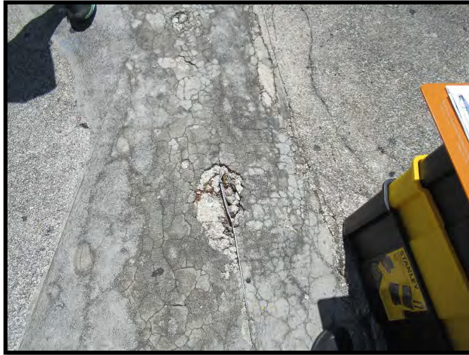
Figure #4: Floor concrete (PPG-03)
