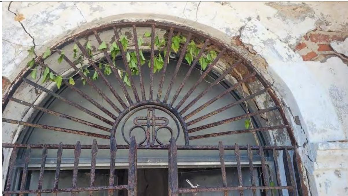
40.2 Entrance arch to the mausoleum. Bricks in walls are visible along with deteriorated metal gates.
