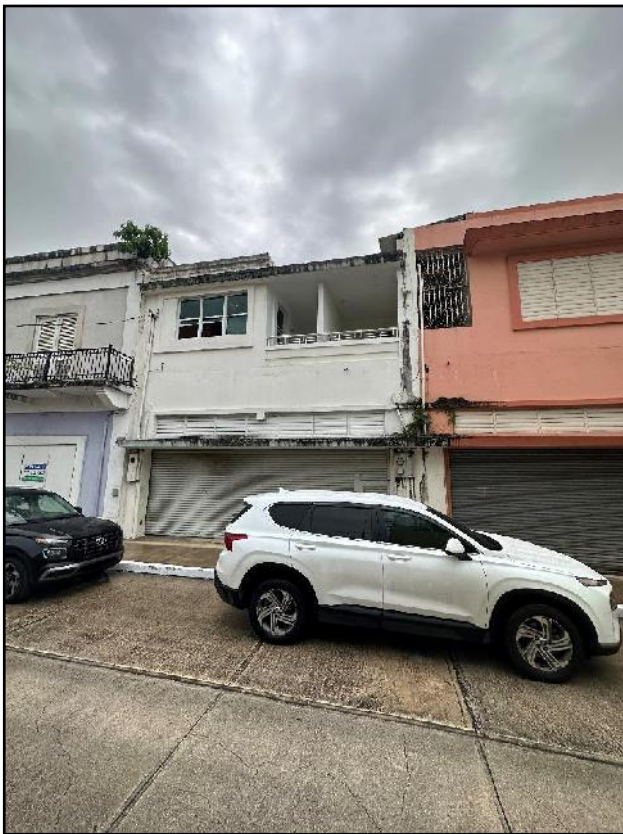
#39 McKinley St. 1 st Floor Exterior Front Facade White Ceramic Tiles Painted with LBP 2 nd Floor Exterior Front Facade White Concrete Walls Painted with LBP
