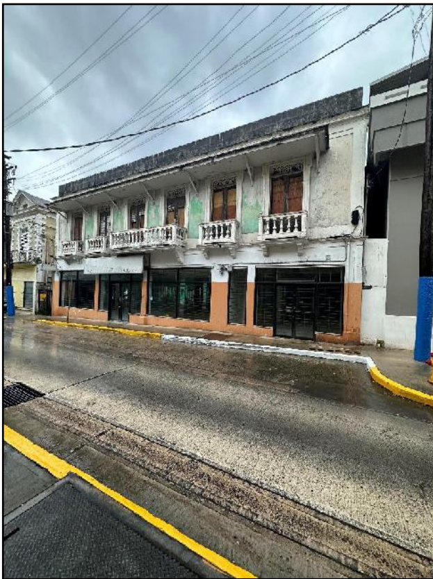
#30 McKinley St. 1 st Floor Exterior Front Facade White & Brown Painted Ceramic Tiles on Walls and Column. White Balcony Ceiling and Joist Painted with LBP 2 nd Floor Exterior Front Facade White Wood Wall and Concrete Column, Concrete White and Green Walls; Balconies Wood Door Frames, and Concrete White Decorative Columns Painted with LBP
