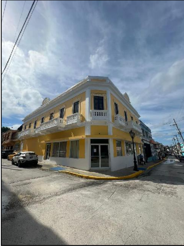
#75 McKinley St. 2 nd Floor Exterior Front Facade Balcony White Concrete Decorative Block Painted with LBP
