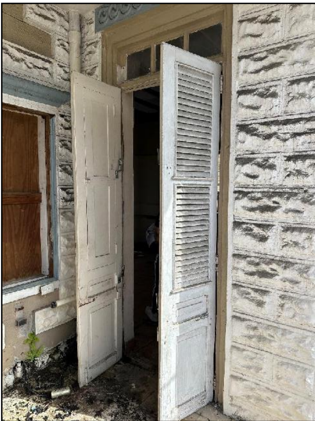
#28 McKinley St. 2 nd Floor Exterior Front Facade Balcony White Decorative Fascia White Wood Door and Frame Painted with LBP
