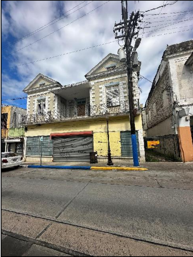
#28 McKinley St. 1 st Floor Exterior Front Facade Lower Walls Ceramic Tiles Painted with LBP
