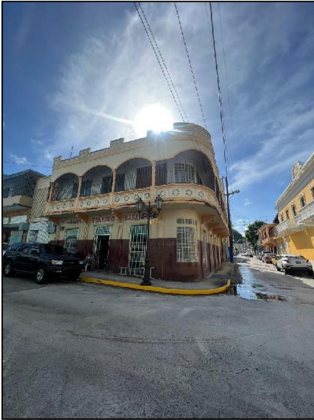
#77 McKinley St. Exterior Front Façade Cream & Brown Concrete Walls Painted with LBP
