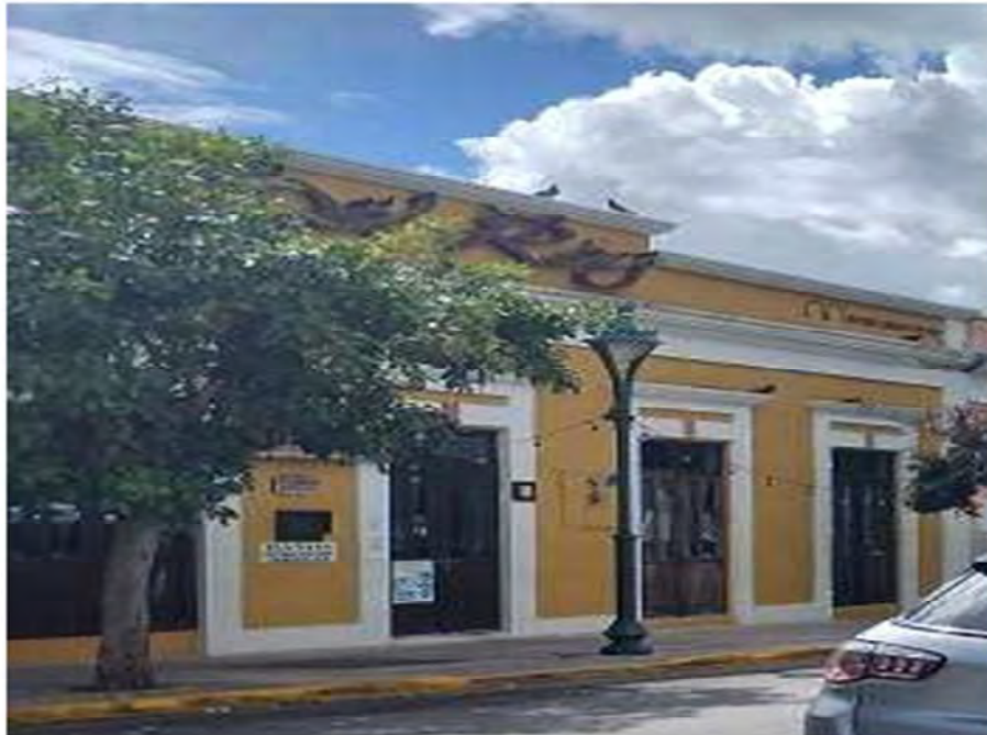
Figure #20: Building identified on map as #2 on Figure #9 on Page #14. Building with cadaster #366-029-037-03-001. Building (Janellys Kitchen) with Neoclassical architectural features. Located on #78 Comercio Street in Juana Diaz.
