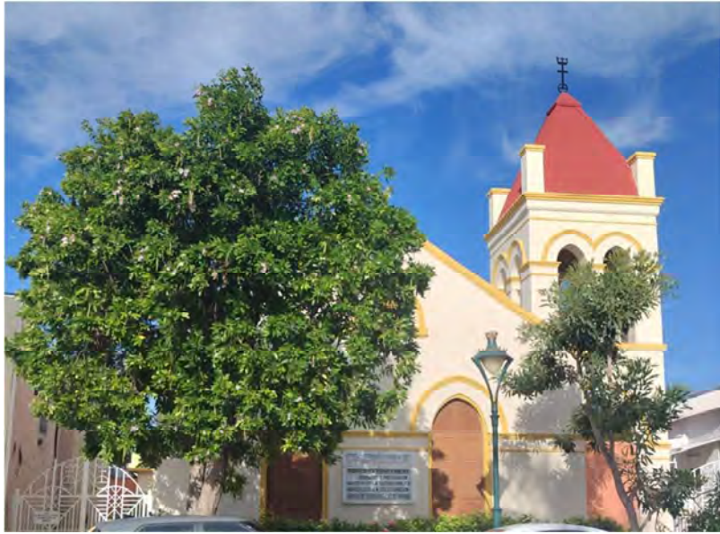
Figure #27: Building identified on map as #9 on Figure #6 on Page #14. Building with cadaster #366-029-024-06-000. Building (Church) of the XX century, located on #11, Carrion Maduro Street in Juana Diaz.
