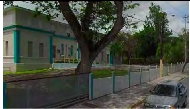
Exterior South Perimeter Fence of the Building
