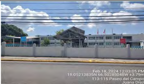
North Facade and Perimeter Fence of the Building
