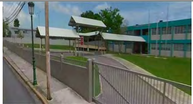
North Facade and Perimeter Fence of the Building (West to East angle)
