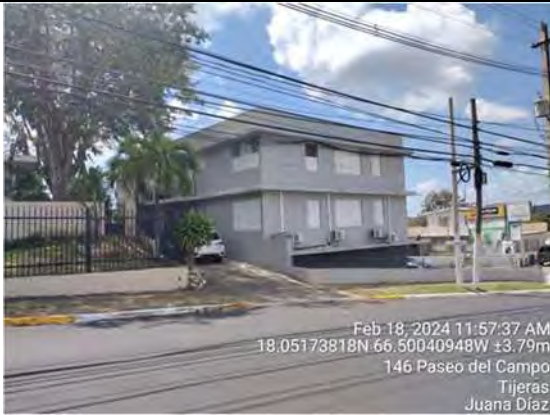
East and North Facade
